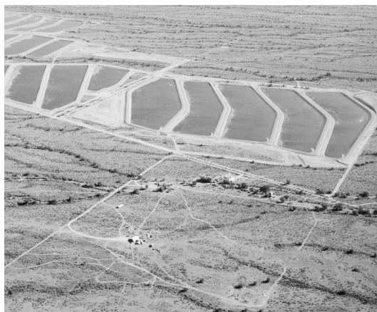
FIGURE 2. CAWCD's Tonopah Desert Recharge Facility looking northeast. The CAP canal which delivers the recharge water to the facility is in the background (arrow). (Photo courtesy of CAWCD)
