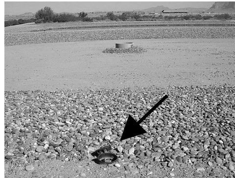
FIGURE 5. Looking north into Basin 5 at the Superstition Mountain Community Facility District #1 Recharge Facility. The flow control valve in the foreground (arrow) controls flow into the vadose zone well seen within the basin in the background of the photo. (Photo by ADWR, 2006)
