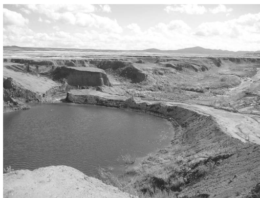
FIGURE 9. Town of Prescott Valley Upper Agua Fria Constructed Recharge Facility. Looking downstream at a berm located in the constructed in-channel recharge facility. The arrow indicates where the end of the berm is located which allows water to flow past and on down to the next berm.
