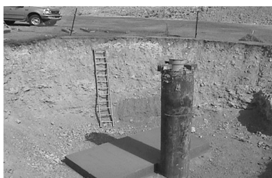
Photo 1. Well and concrete pad prior to vault placement.
