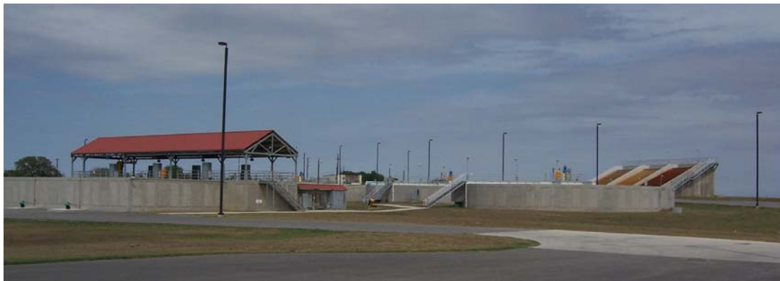
Figure 3-3: Water treatment plant (Morris, 2006)
