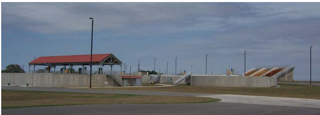
Figure 3: Water Treatment Plant (Morris, 2006)
