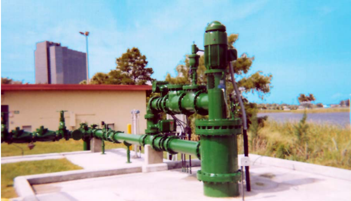
Figure 1-1. A typical ASR well (courtesy of CH 2 M Hill, Inc.)
