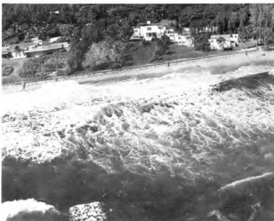
FIG. 11. WAVE ACTION ON CHECKER-BOARD REVETMENT, JUPITER ISLAND, FLA.
