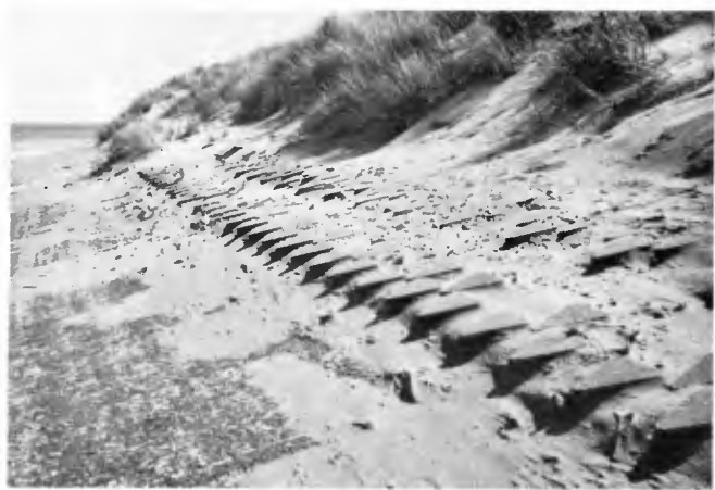
FIG. 8. SAND DEPOSITS ON REVETMENT OF FIG. 7 (TEXEL)
