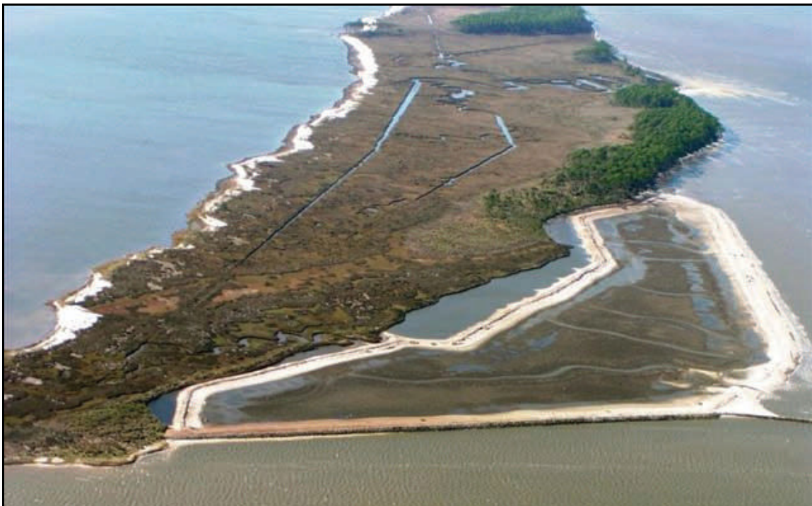
Figure 17. Completed Deer Island Marsh Project (Ramseur, 2010).
