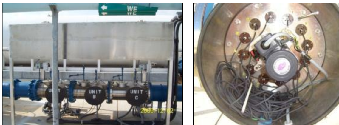
Figure 6-6 -- The UV disinfection units. Units are arranged in series (left), and a cross-section view of a single unit showing 12 UV lamps oriented perpendicular to flow direction (right).
