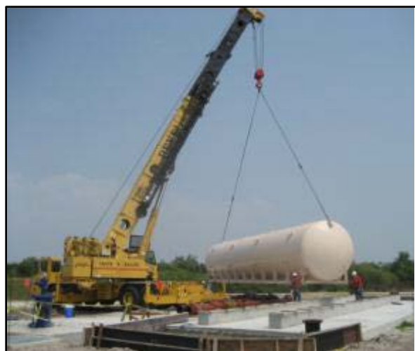
C. Installing the pressure filter.
