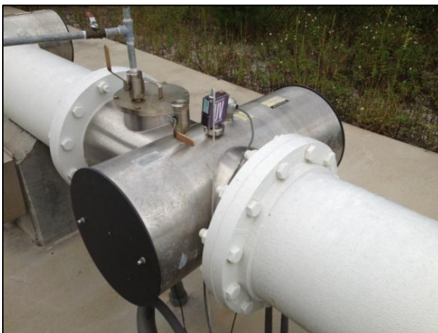
Figure 6-16 -- A single chamber of the UV disinfection unit.
