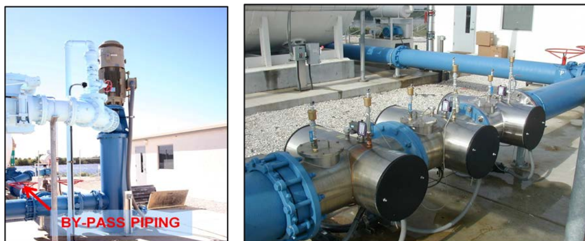
Figure 8-6 -- Completed by-pass piping (left), completion of 3-unit, in-line UV disinfection system (right).
