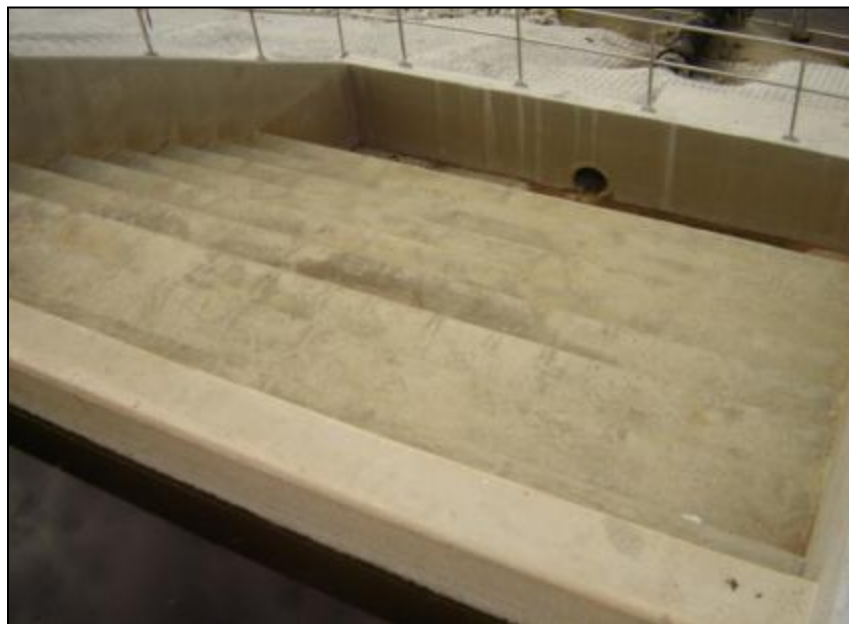
Figure 6-10 -- The spill structure and cascade aerator.
