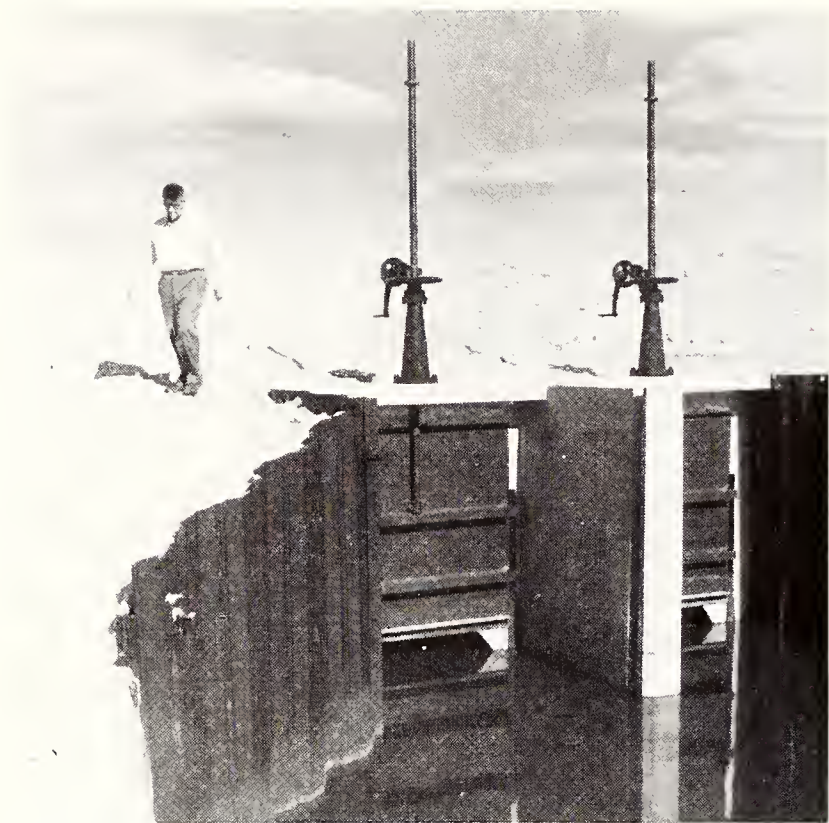
These gated culverts provide facilities for passage of water through a main levee as conditions demand for local water control.
