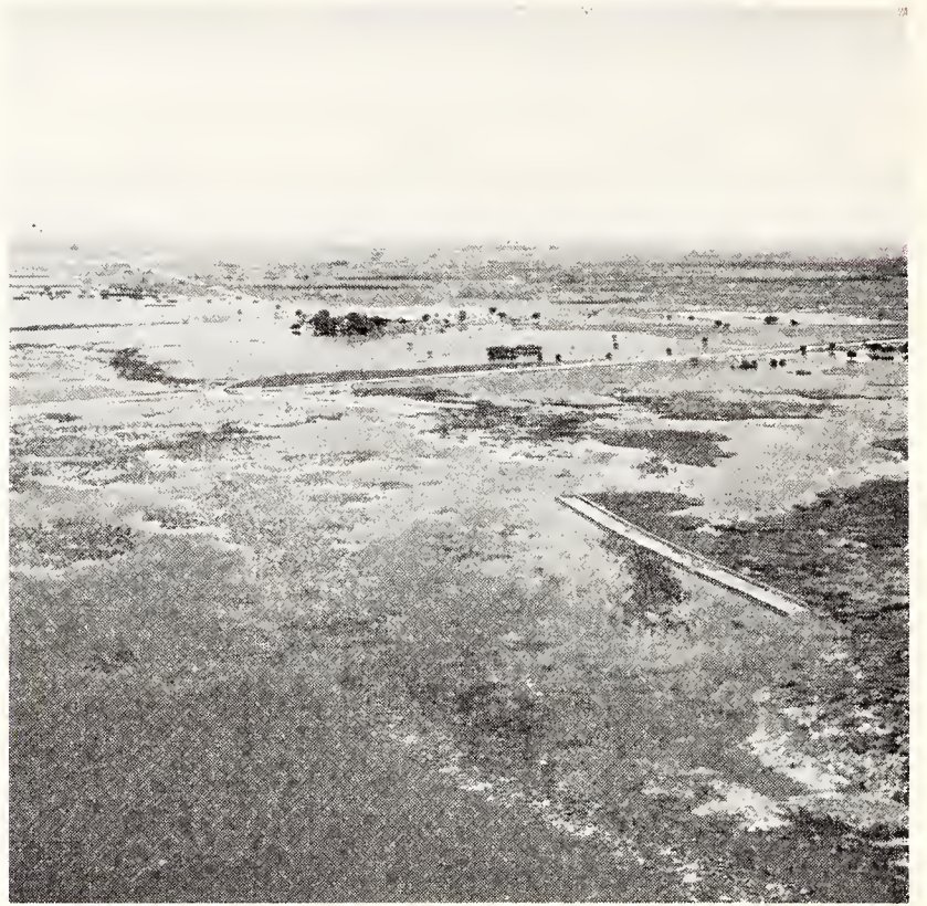
This highway bridge across the Kissimmee River on State Road 60 washed out and broke apart during high water in 1953.
