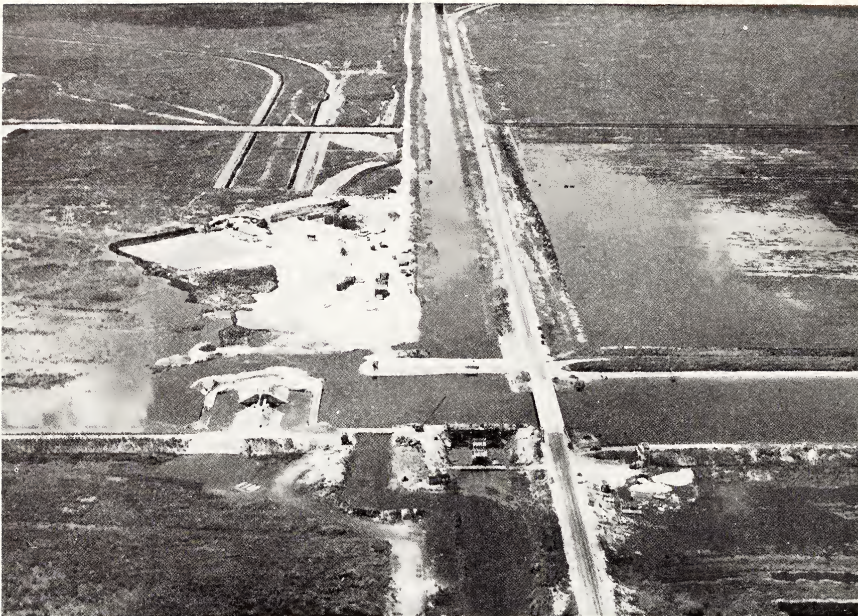
A major control unit under construction at 20-Mile Bend, just west of West Palm Beach. This unit involves a spillway, gated culverts and a pumping station located at the intersection of several major canals and the northern-most conservation area.
