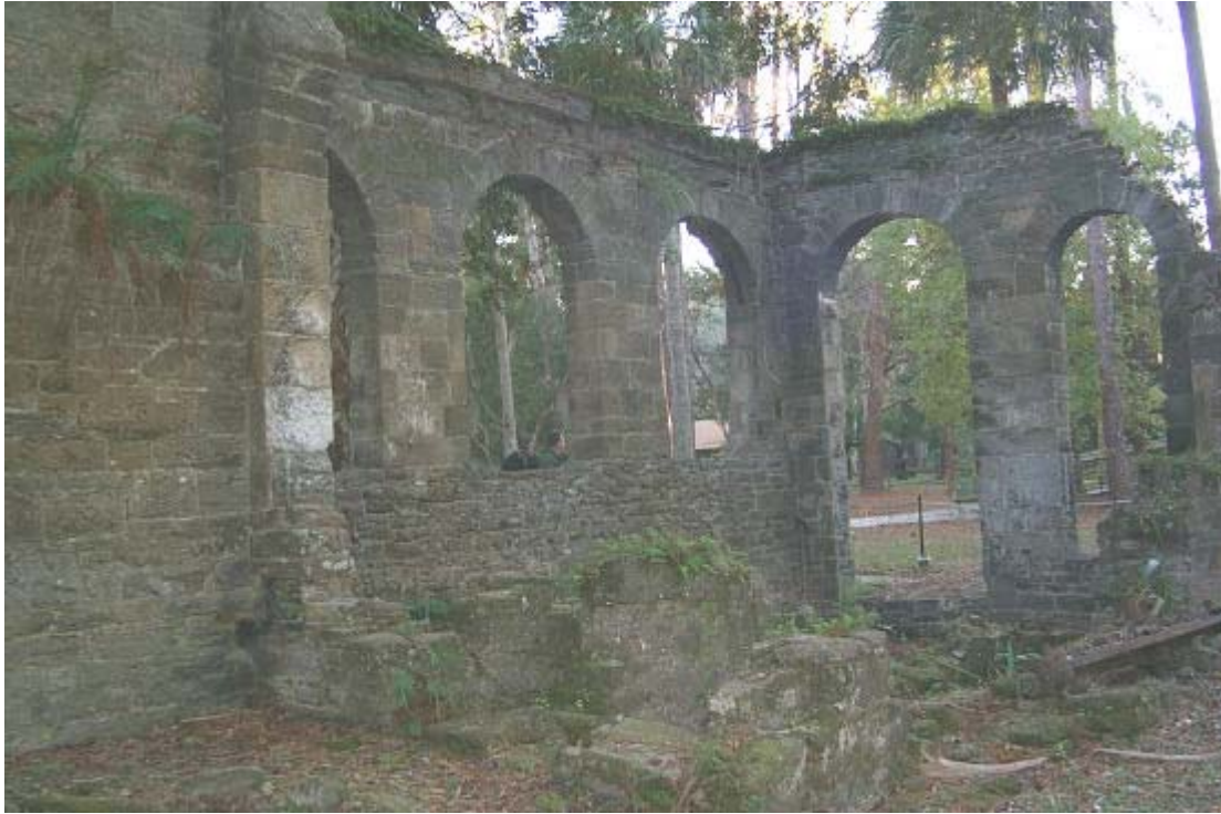
Figure 5. Ruins of New Smyrna Sugar Mills (1830). (Photo courtesy of the author.)
