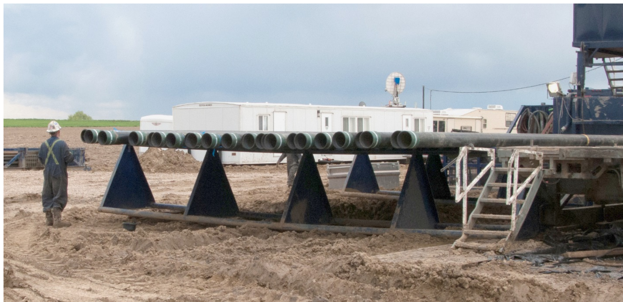
Figure 3-8. Sections of well casing ready for installation at a well site in Colorado.
