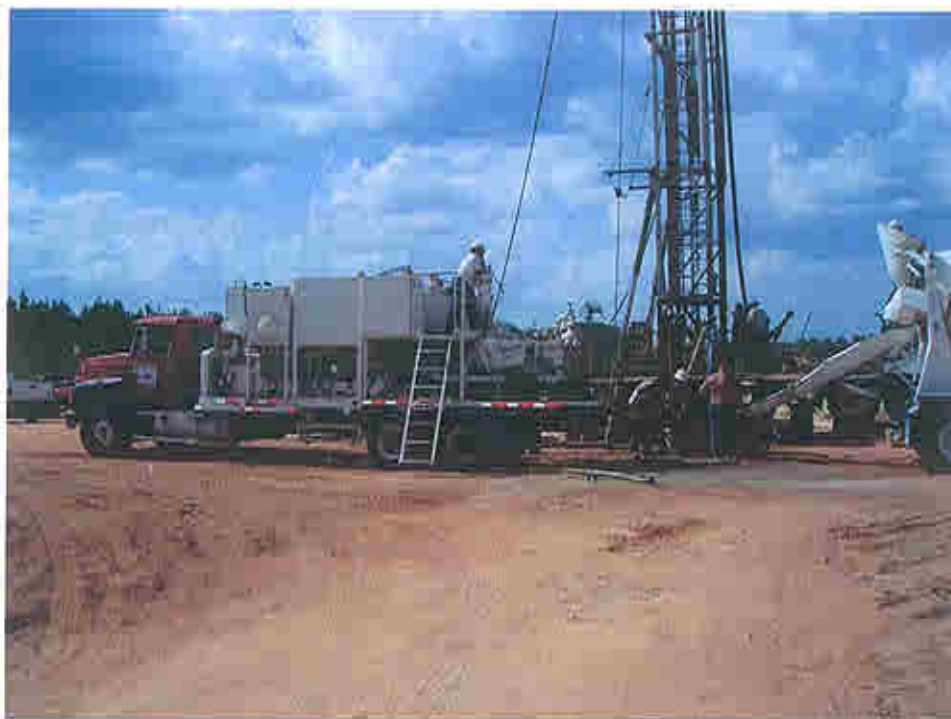
Photograph D-5- Cementing Operation
