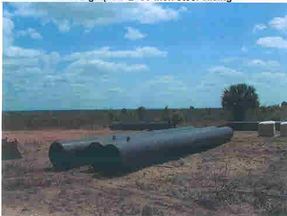
Photograph D-2- 36-inch steel casing
