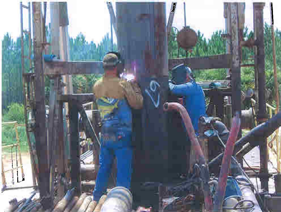
Photograph D-8 - Welding 24-inch casing
