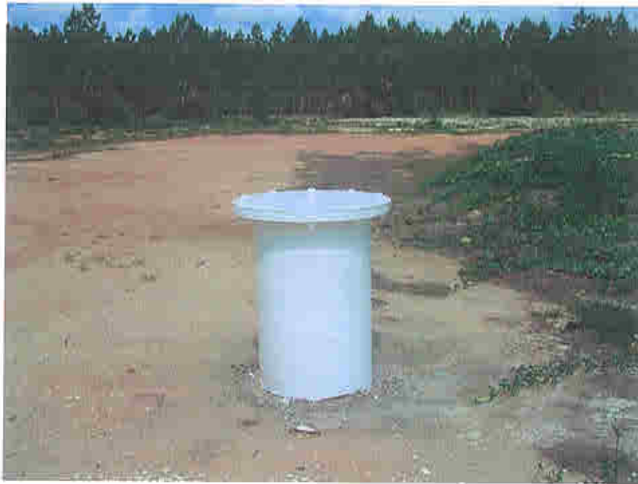
Photograph D-19 - HH-1 Wellhead Completion
