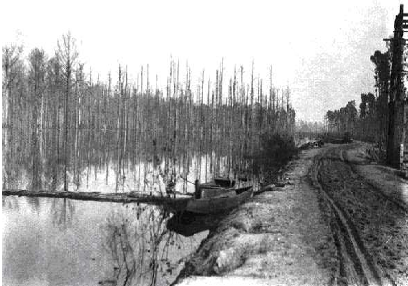
Photograph 6 Merritt's Mill Pond Dam (1922) Merritt's Mill Pond Arsenic Study Marianna, Jackson County, Florida
