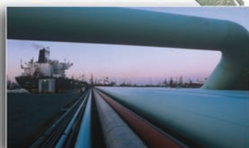
Pipe conveyor oil, Mexico.
