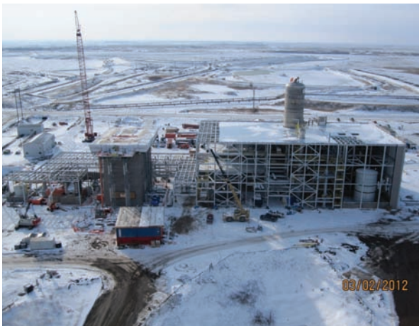
General view of the 1 megatonne/year CO 2 capture plant under construction at the SaskPower Boundary Dam Generating Station near Estevan, Saskatchewan, Canada. (Courtesy: SaskPower)
