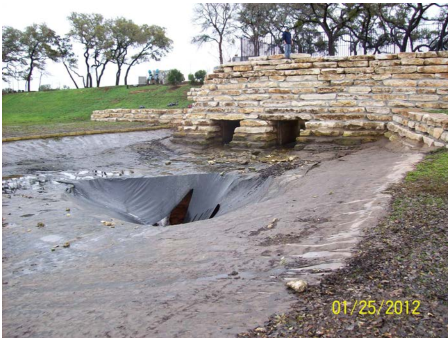
Sinkhole collapse under an engineered pond in Austin, Texas.
