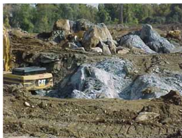
Figure 4. Typical excavation in karst
