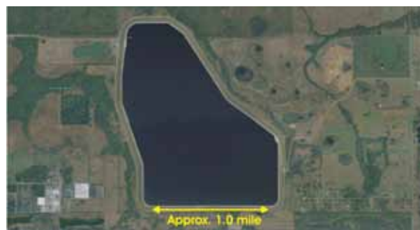
Figure 1. C.W. Bill Young (Tampa Bay Regional) Reservoir site, Hillsborough County, Florida. Aerial photograph from Google Earth (2017).
