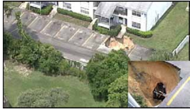
Figure 2. Bordeaux Apartments sinkhole, Tampa, FL, aerial photo showing car being swallowed by a sinkhole.
