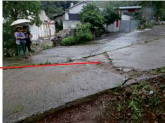
Figure 8. An example of ground subsidence points identified by InSAR data
