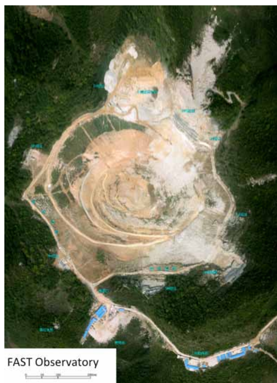
Figure 4. Aerial view of the Dawodang depression during the construction of FAST, image was taken by a DJI drone (Mar 31, 2012).
