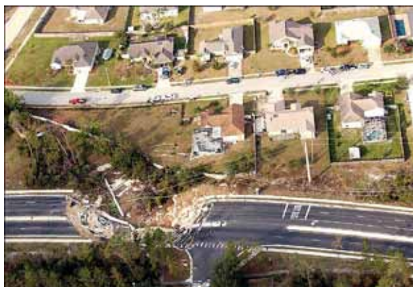
Figure 8. Site 2 sinkhole, top of photograph is north (New York Times, 2004)
