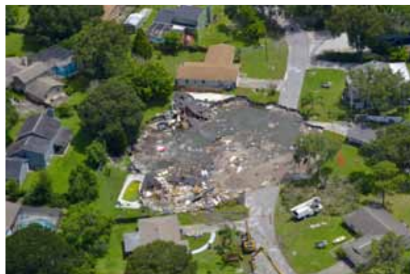
Figure 1. Ocean Pines Drive sinkhole, bottom of photograph is north (WFLA NBC 8, 2017)
