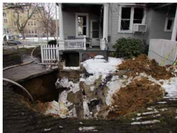
Figure 1. The sinkhole created by water used to fight the fire.
