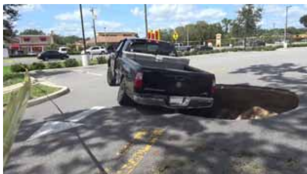
Figure 14. Site 3B sinkhole, top left of photograph is north (Kenyon, 2017).
