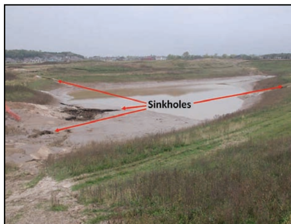
Figure 2. Sinkholes in Dancing Water Pond, Woodbury, Minnesota (looking southwest). Picture taken October 12, 2005 by E. C. Alexander, Jr. Long axis of left sinkhole (longest arrow) is approximately 9 m.
