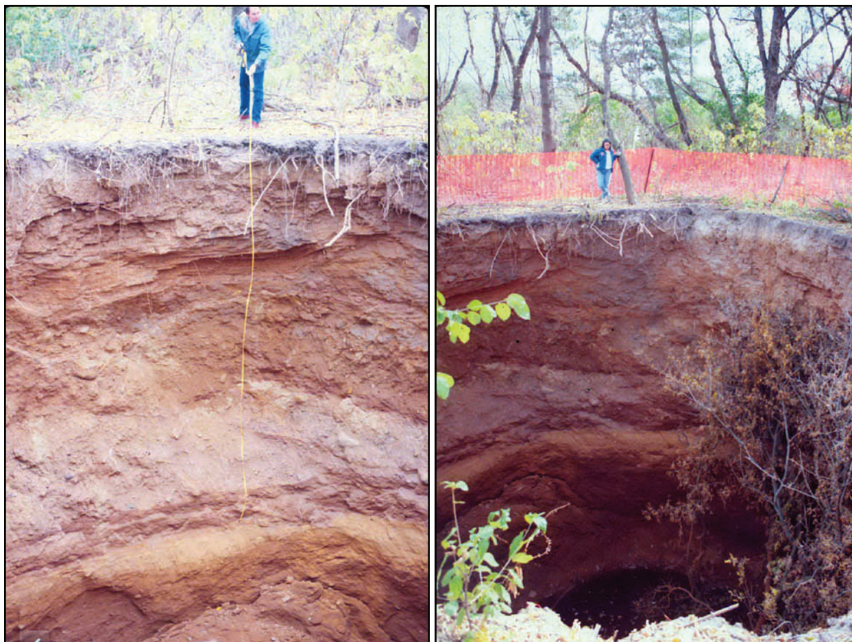
Figure 7. Collapse structure, Mahtomedi, Minnesota. Both 7A (left) and 7B (right) show the glacial till walls of the collapse. Note the small tree in 7B (right) that dropped into the collapse. Photos from D. Setterholm.
