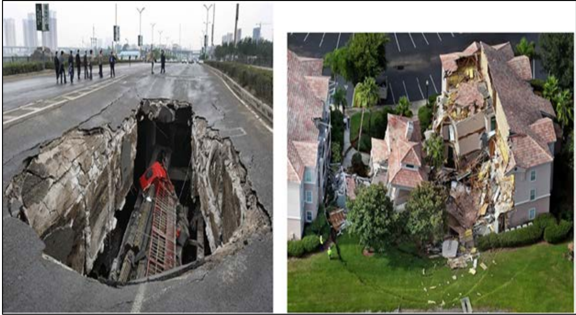
Figure 2.7. Bridge and building collapses caused by sinkhole collapse ( http://www.amusingplanet.com/2013/09/disastrous-sinkholes )
