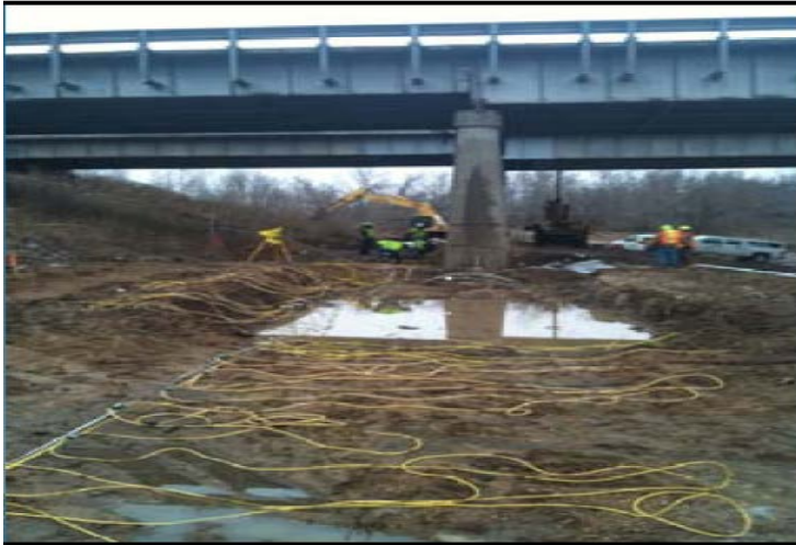
Figure 7.4. Data acquisition under the bridge at the project site
