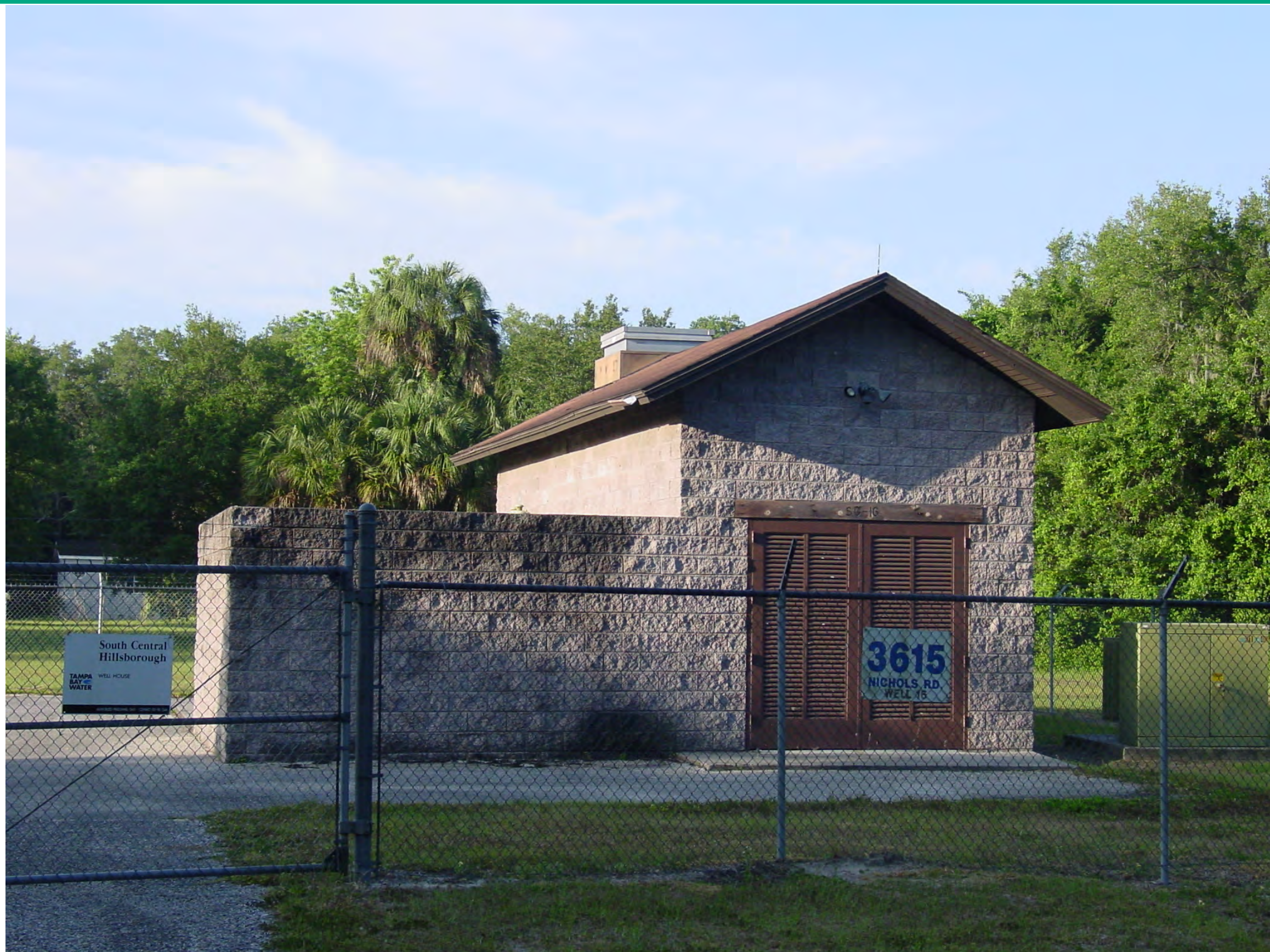
Photograph 4 Tampa Bay Water South Central Hillsborough Regional Well Field Pump House (SC-15) Pritcher Road Environmental Assessment Lithia, Hillsborough County, Florida
