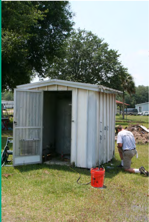
Bryant Mobile Home Park Supply Well
