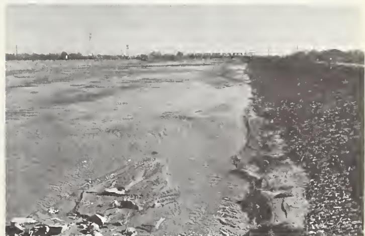
FIGURE 9.— Straight reach of lower Los Angeles River where handplaced stone withstood the flood. Note bridge truss destroyed in upper photograph.
