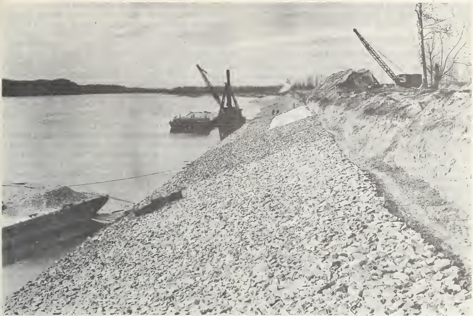
FIGURE 12. — Paving for bank protection.
