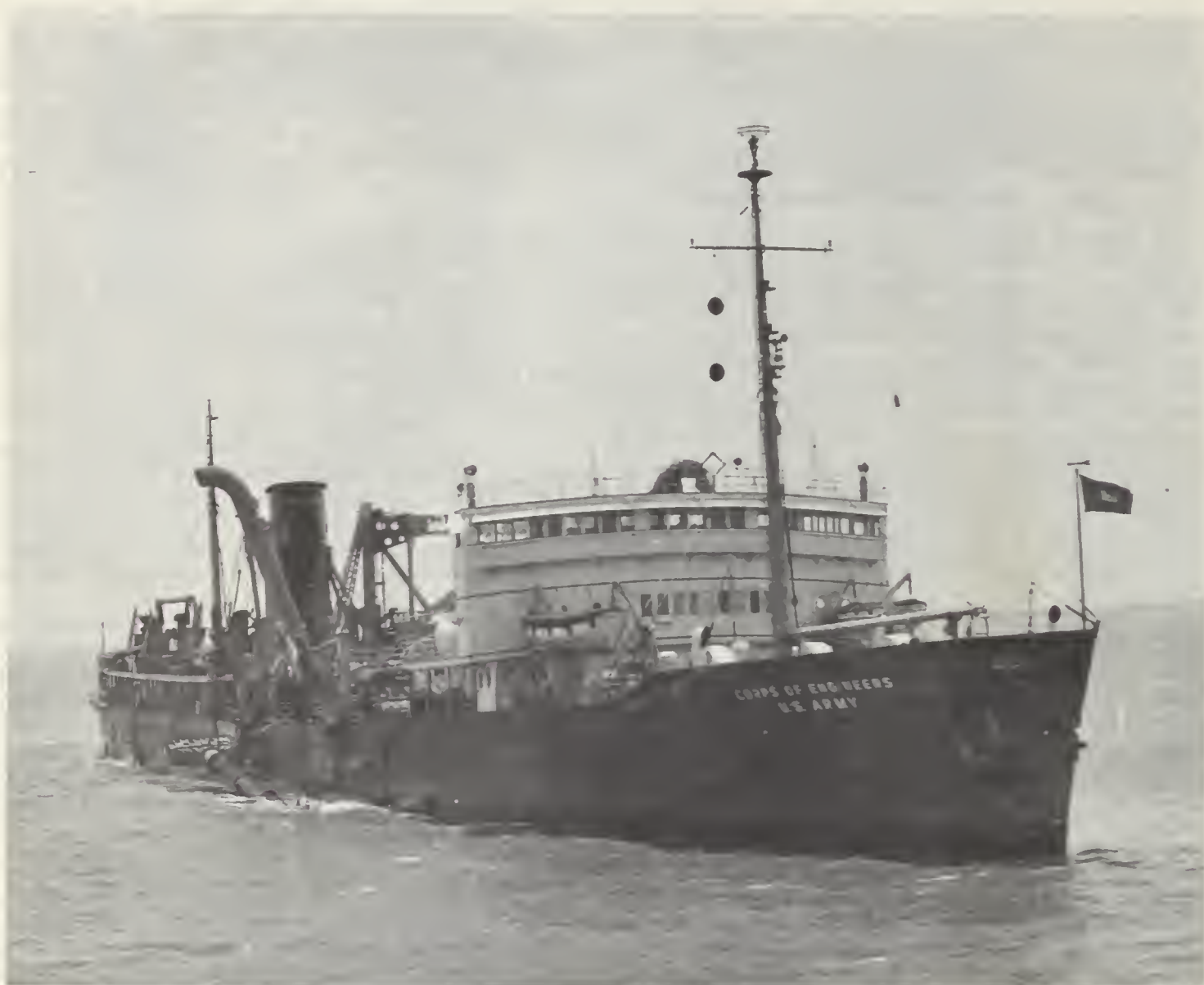
FIGURE 7. — Hopper dredge Goethals , showing 42-inch discharge pipe for sump rehandling.
