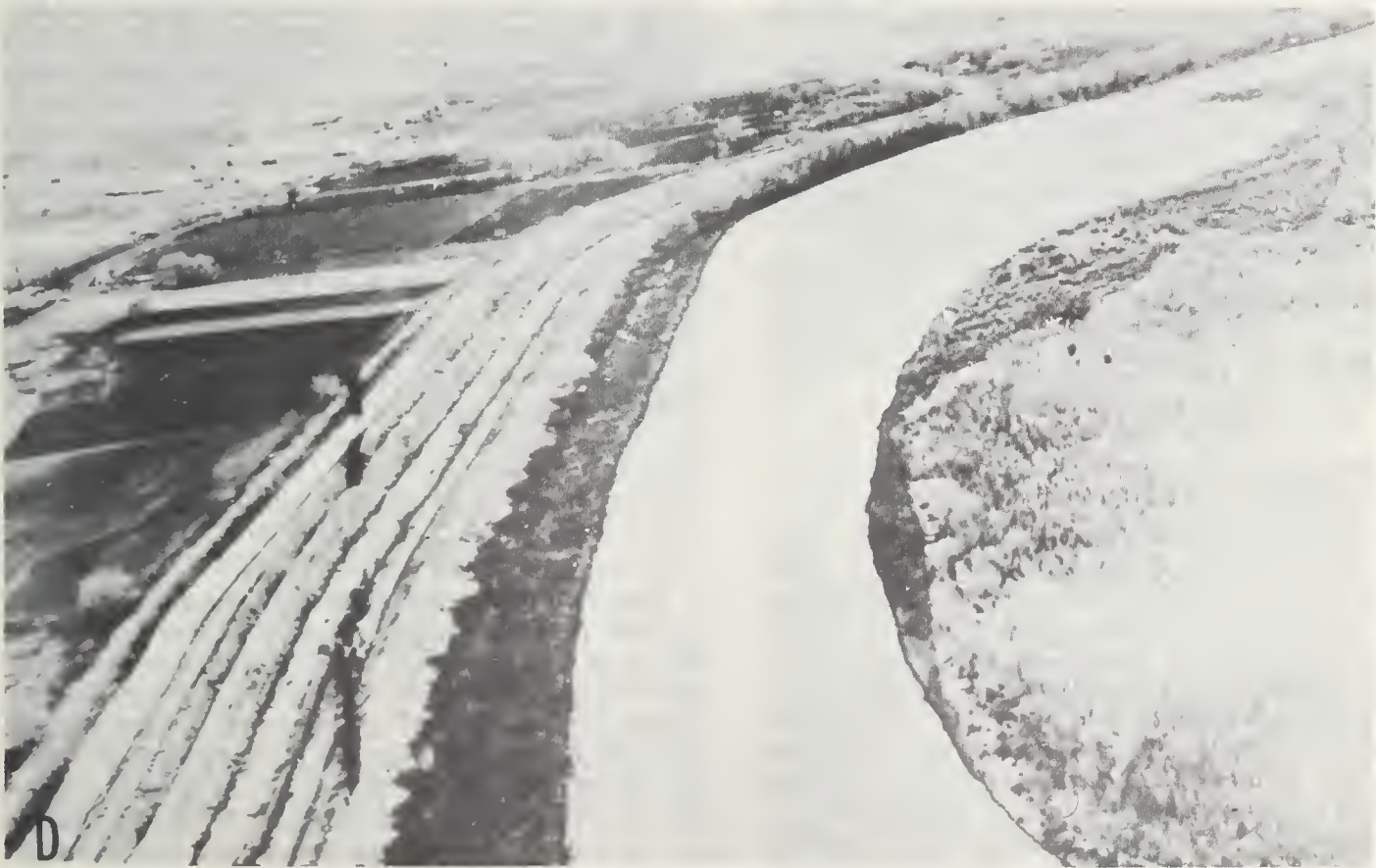
jetty field in June 1953; C , September 1955, about 2 years after completion of emergency work; D , April 1958, about 5 years after completion of bank protection works.
