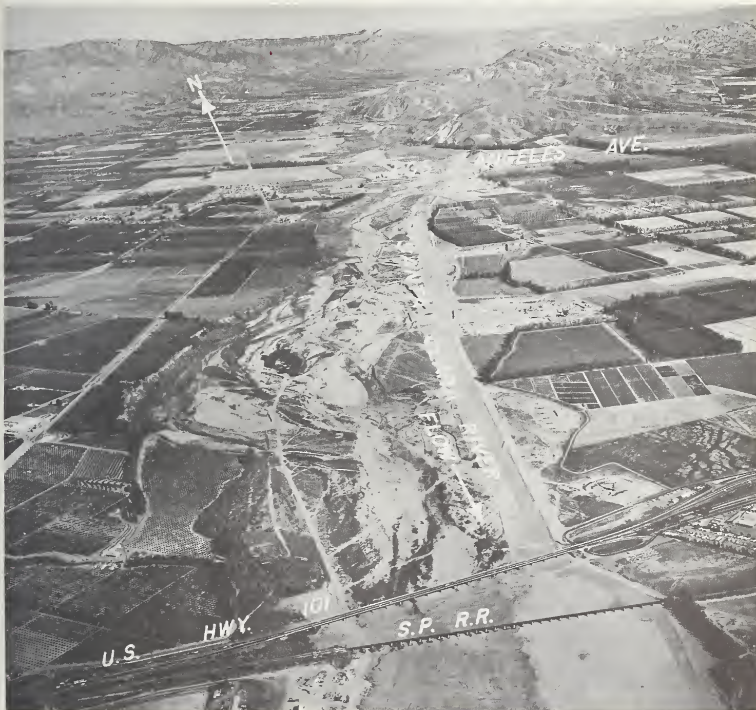
FIGURE 20.—Upstream view of Santa Clara River in Ventura County, Calif., showing a single levee designed to confine a discharge of 225,000 c.f.s.
