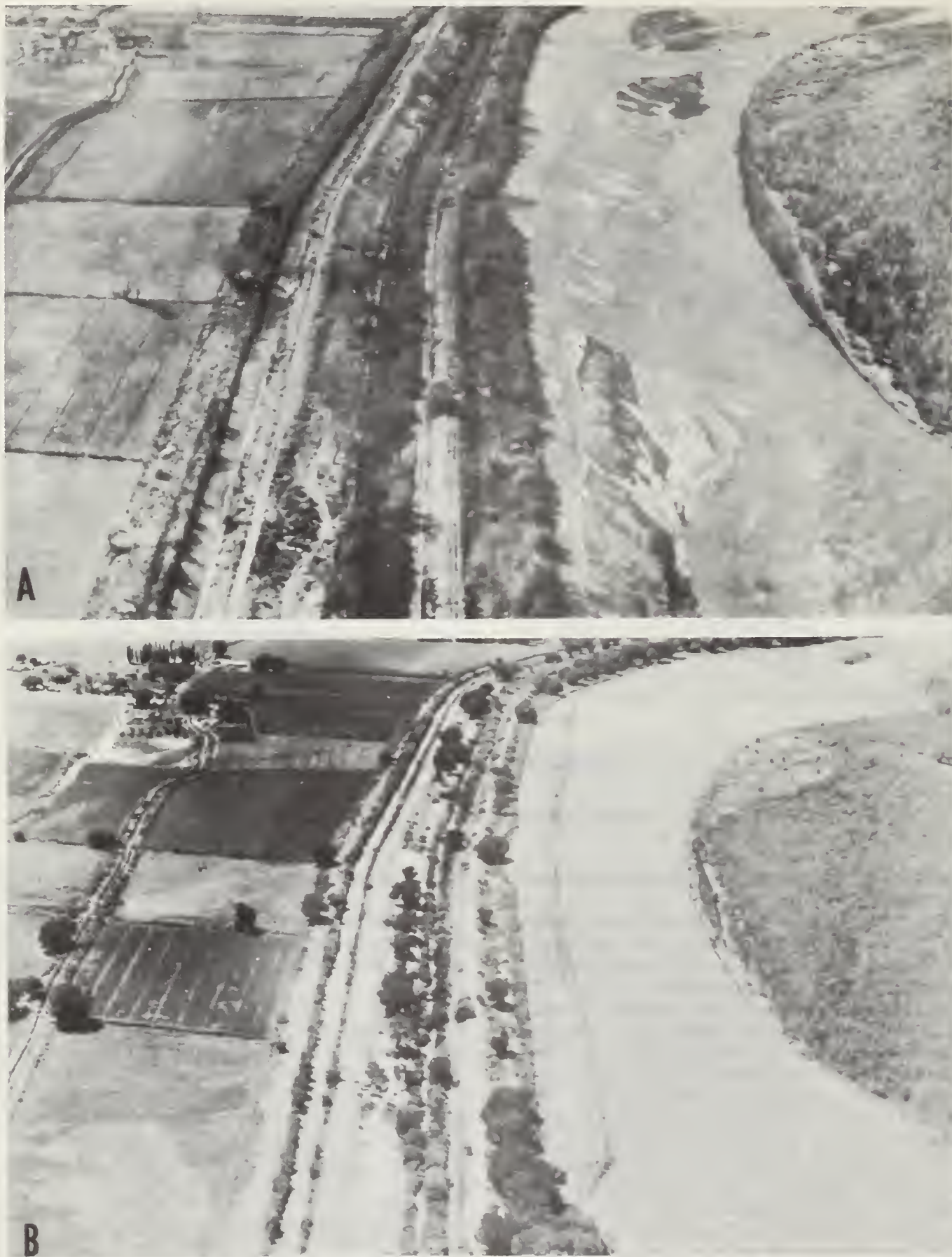
FIGURE 5. — Emergency flood control work on Rio Grande near Bernalillo: A , December 1952, looking downstream prior to installation of bank protection works; B , August 1953, at the same location after installation of Kellner
