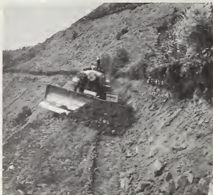
FIGURE 9. — The trench is constructed along the platform by a cut-and-fill operation. With the use of full angle and tilt of the blade, excavated dirt spills under the outer track of the machine, where it is packed to form the outer dike of the trench.
