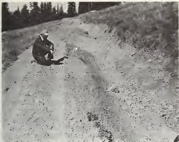
FIGURE 11.— Completed trench after construction of cross dams or baffles. Trench has a storage capacity of 7 to 10 cubic feet per lineal foot of trench. Cross dams are lower than trench dike, to allow equalization of stored water in trench and to prevent spill over the trench.
