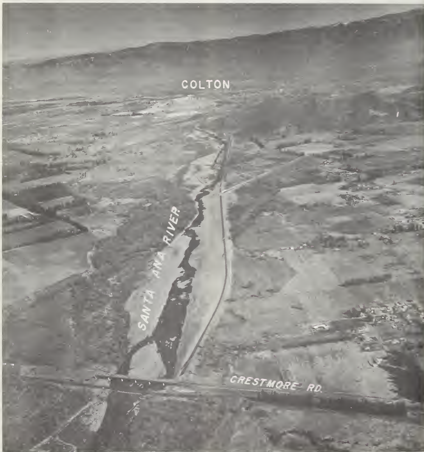
FIGURE 17. — Upstream view of Santa Ana River in Riverside County, Calif., showing partial completion of the project. Double levees were subsequently built downstream from Crestmore Road to confine a discharge of 195,000 c.f.s.
