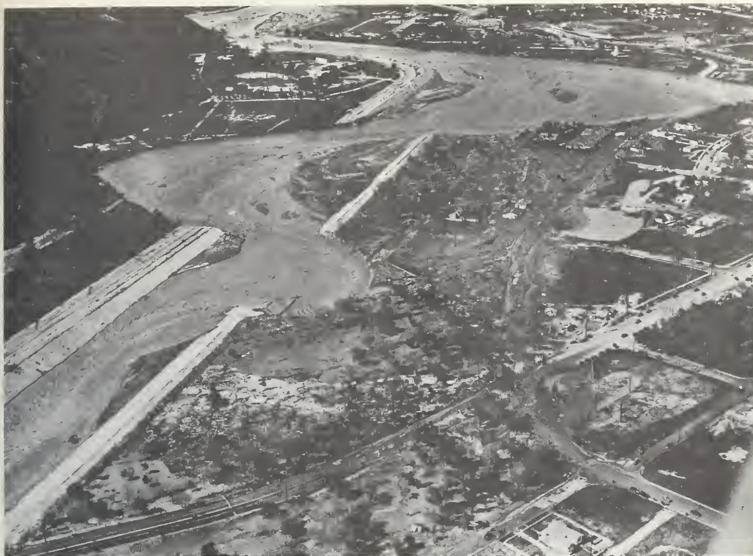
FIGURE 5.— Upstream view of damage to Los Angeles River channel in 1938 flood: Maximum discharge 60,000 c.f.s.; maximum velocity about 20 f.p.s.
