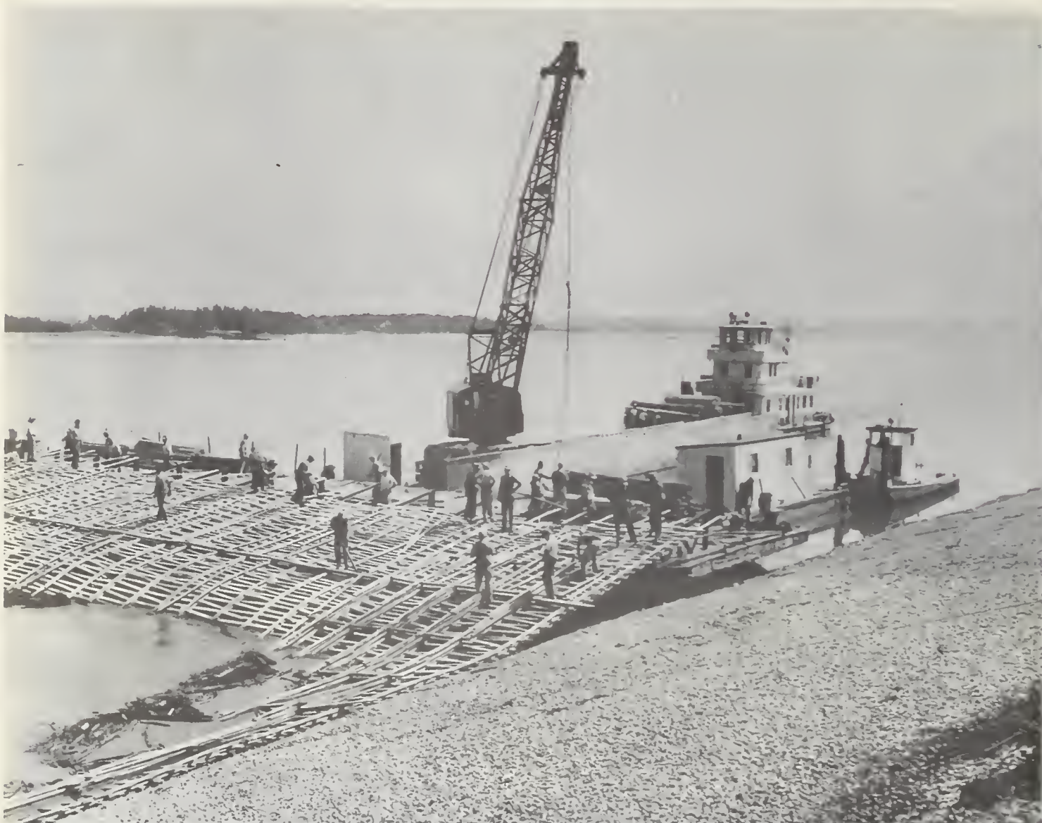
FIGURE 11. — Woven mattress for bank protection.
