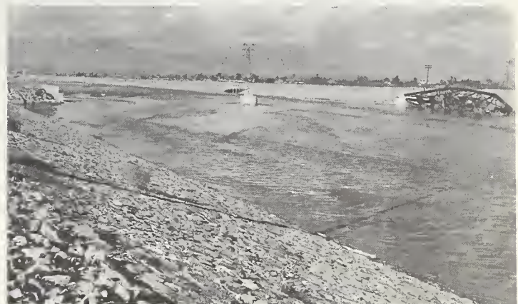
FIGURE 8.— Downstream views of Los Angeles River showing bank failure after dump stone was undercut and washed away.
