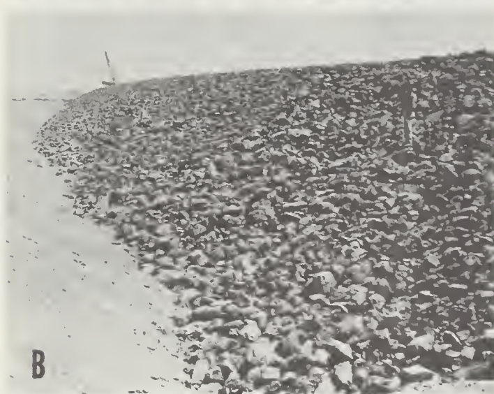
FIGURE 23. — Downstream views of levee construction on Santa Maria River: A, General view showing toe trench excavation; B, closeup view of riprap revetment.
