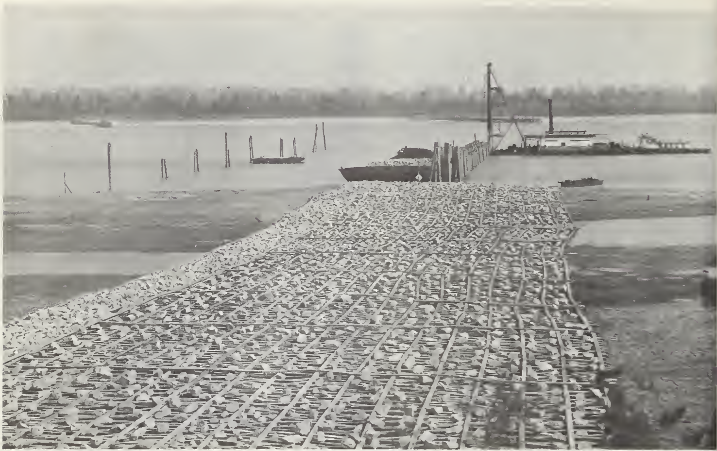
FIGURE 6. — Mattress and paving for piling dikes under construction.
