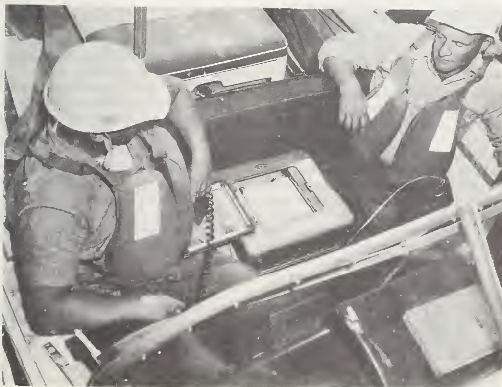
FIGURE 11. — Survey crew and equipment.
