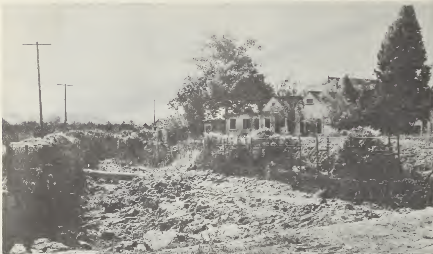
FIGURE 4. — Typical pipe-and-wire fence used for bank protection. Note how channel bottom is eroding and undercutting fence along left bank.
