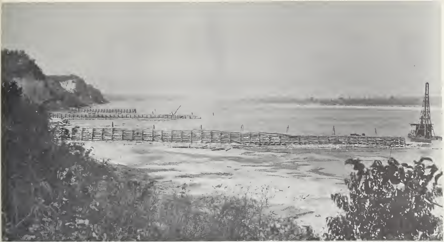
FIGURE 9. — Crib dike under construction.
