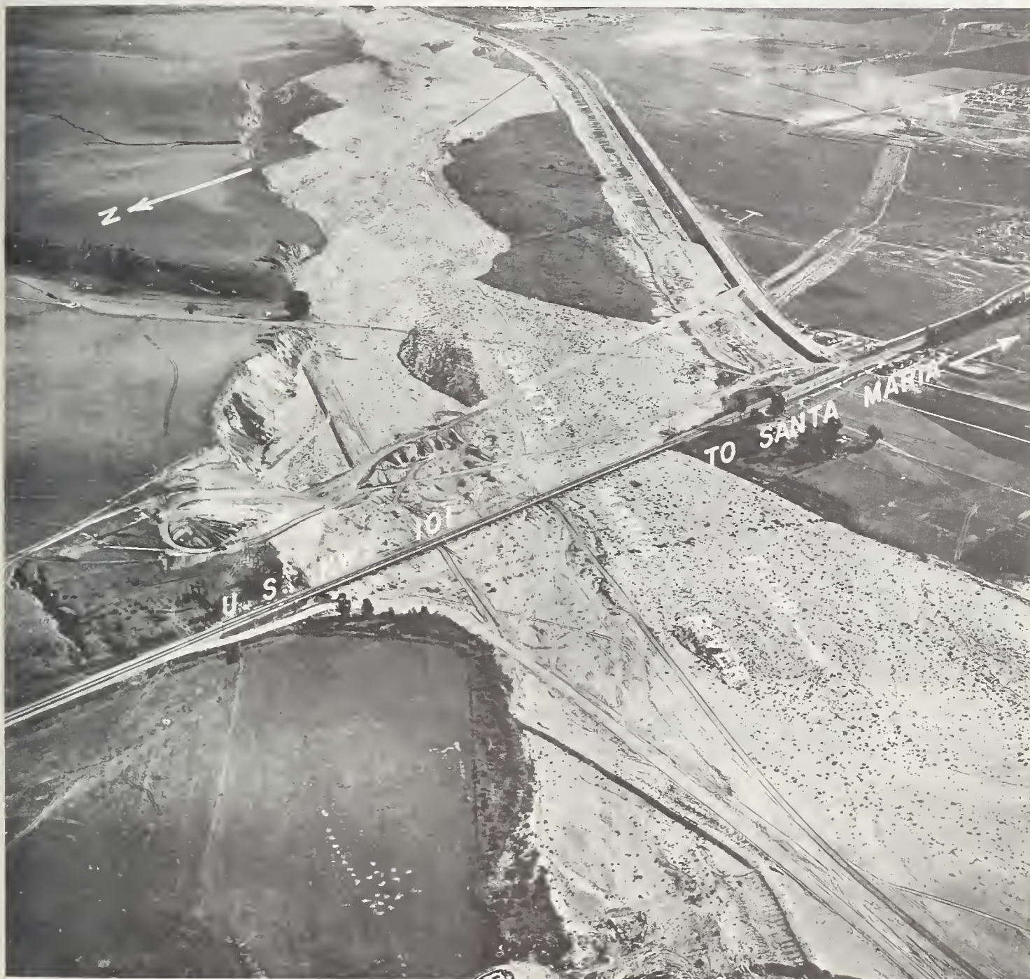
FIGURE 22.—Upstream of Santa Maria River in Santa Barbara County, Calif., showing partial completion of the project. Right and left bank levees were subsequently built downstream from U.S. Highway 101 to contain 150,000 c.f.s.
