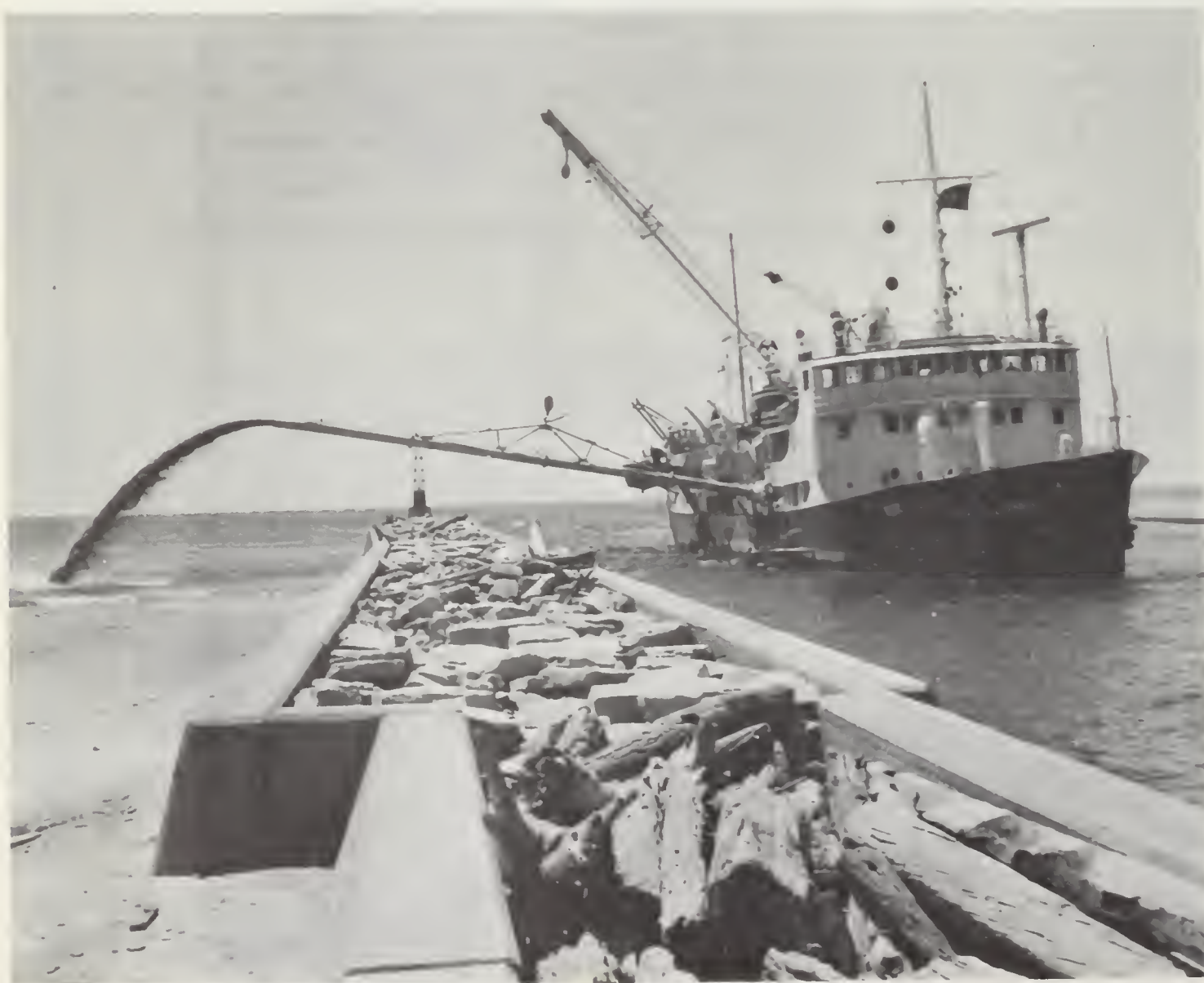
FIGURE 12. — Hopper dredge Hains during side-casting operations at White Lake Harbor, Mich.
