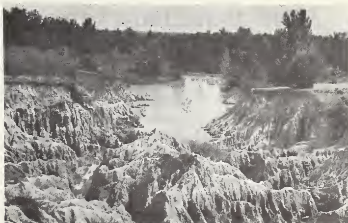
FIGURE 7. — Process of gully stabilization by the construction of a dam (in background) and the planting of bermudagrass (in foreground).
