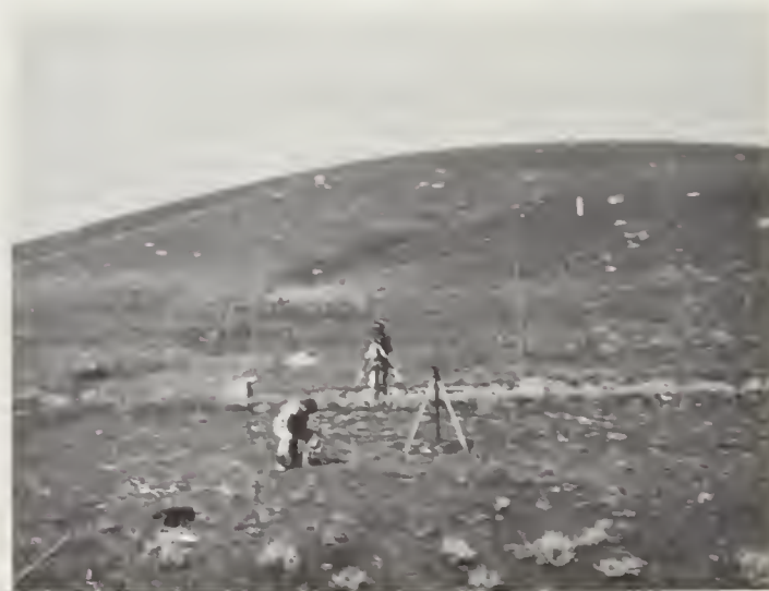
FIGURE 11.—Typical arrangement of Raydist shore station units at Garrison Reservoir.
