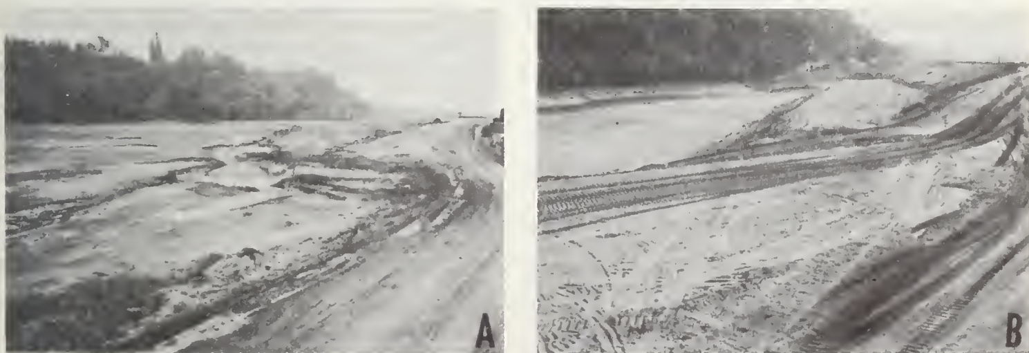
FIGURE 1.— Puddingstone diversion dam after 1961-62 storm season (A) and after debris was removed (B).
