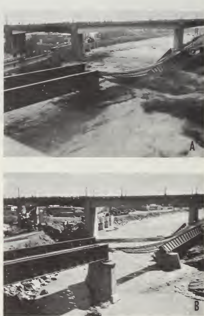
FIGURE 7.—Railroad bridge crossing Los Angeles River destroyed during 1938 flood as result of underscour of pier: A , High discharge during flood; B , after flood receded.
