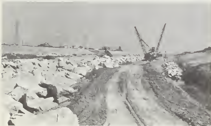
FIGURE 14. — Eroded streambed in vicinity of stabilizer: A, Scour at stabilizer for skew railroad bridge is about 6 feet and diminishes to 3 feet in a downstream distance of 80 feet; B, along right levee toe, scour is maximum of 5 feet and diminishes to 3 feet in a downstream distance of 500 feet.
