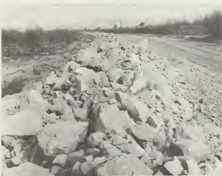
FIGURE 2. — Riprap material on the ground in the form of a windrow.
