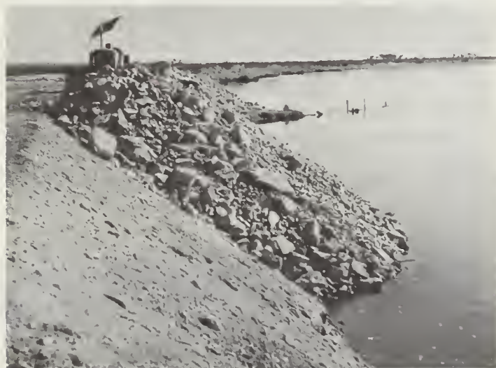
FIGURE 4. — Riprap being placed by bulldozer.
