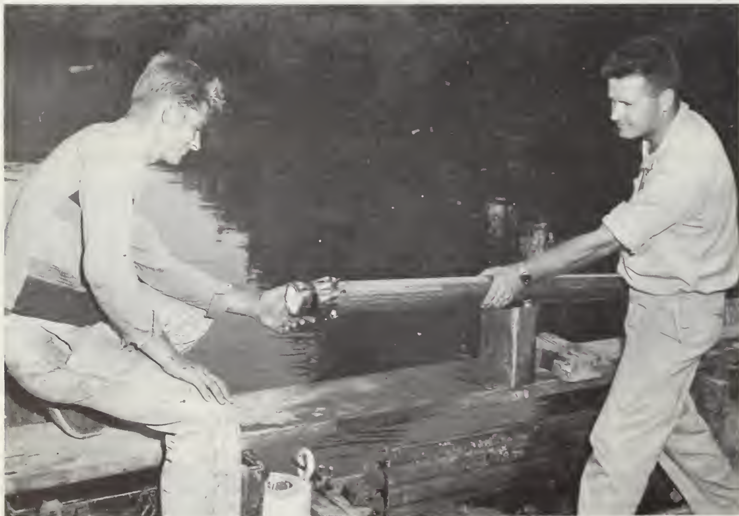
FIGURE 5. — Transferring core from sample tube to plastic storage tube.
