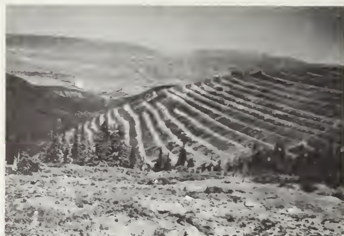
FIGURE 5.—Contour trench system installed on a deteriorated watershed for flood prevention and watershed protection purposes. Slope gradients vary from 30 to 70 percent. Evaluations made subsequent to construction indicate the trenching system has materially reduced downstream sedimentation.
