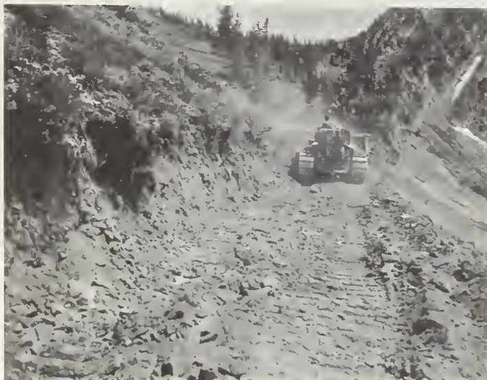
FIGURE 7. — On steep terrain, the first step of contour trench construction is building a level work platform on which the tractor operates. The platform need be no wider than necessary to accommodate the equipment safely.
