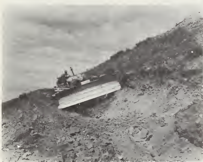
FIGURE 8. — After the platform is constructed, the upper 2 feet of the steep vertical cutbank are knocked down to aid in backsloping.
