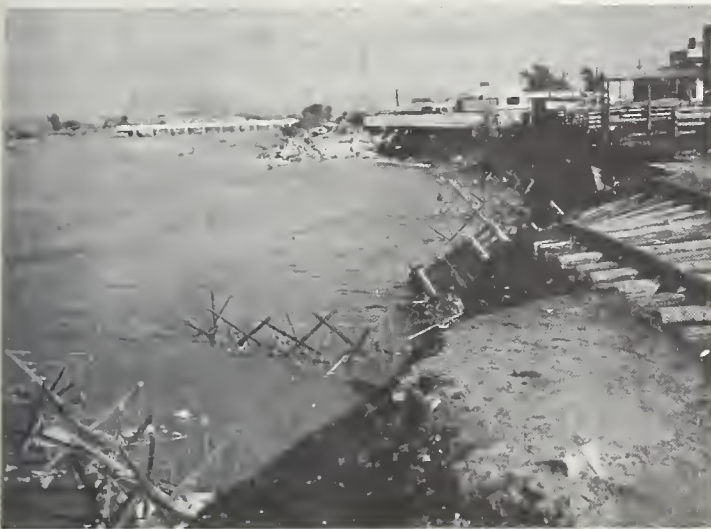
FIGURE 8.— Downstream views of Los Angeles River showing bank failure after dump stone was undercut and washed away.
