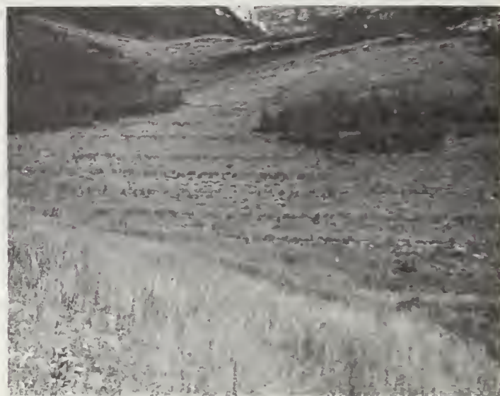
FIGURE 13. — Left, system of contour trenches constructed on Dry Creek flood-source area in fall of 1958. Trenches break up gully pattern. Right, Dry Creek area 3 years after installation of contour trench system (1961). Seeded grasses well established on soils disturbed by construction activities. Improved soil moisture condition between trenches have contributed to reestablishment of native vegetation.
