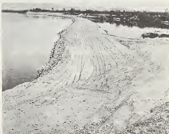
FIGURE 3.—Embankment for bank protection and alinement.
