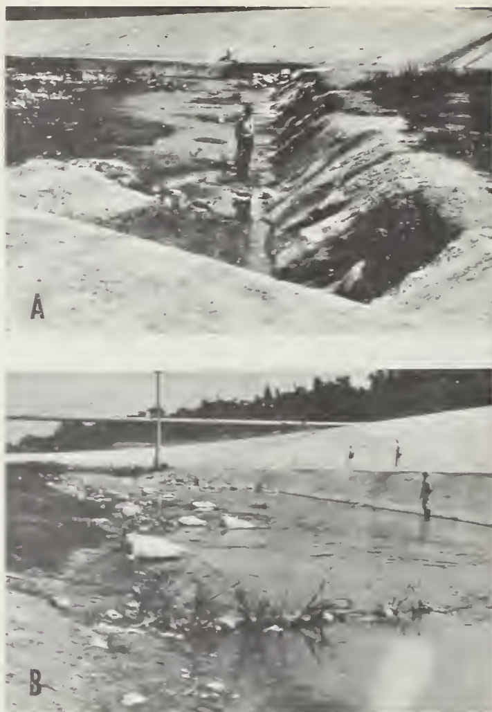
FIGURE 14. — Eroded streambed in vicinity of stabilizer: A, Scour at stabilizer for skew railroad bridge is about 6 feet and diminishes to 3 feet in a downstream distance of 80 feet; B, along right levee toe, scour is maximum of 5 feet and diminishes to 3 feet in a downstream distance of 500 feet.
