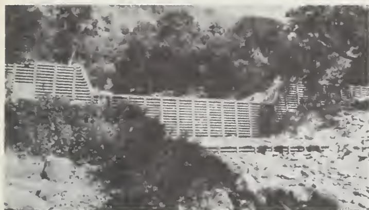
FIGURE 3. — Typical stabilization structures: Left, concrete crib; and right, metal bin.
