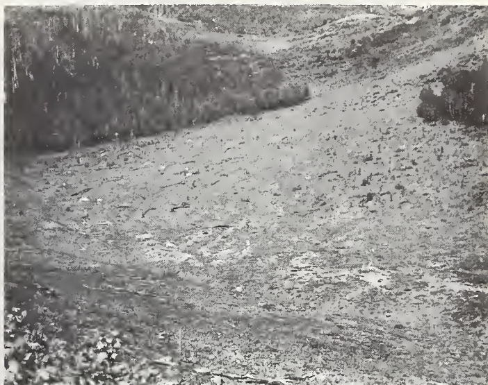
FIGURE 11.— Completed trench after construction of cross dams or baffles. Trench has a storage capacity of 7 to 10 cubic feet per lineal foot of trench. Cross dams are lower than trench dike, to allow equalization of stored water in trench and to prevent spill over the trench.
