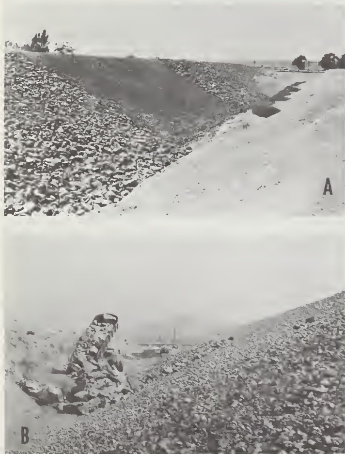
FIGURE 21. — Riprap revetment on Santa Clara River levee: A, Downstream view showing filter course and facing stone; B, upstream view showing placing of heavy stone in toe trench.
