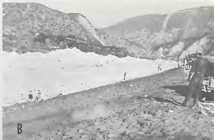
FIGURE 16.—Cobblestones obtained from streambed are graded and placed on levee, then grouted: A, Ventura River levee; B, San Gabriel River levee. Note character of streambed material in toe trench excavation.
