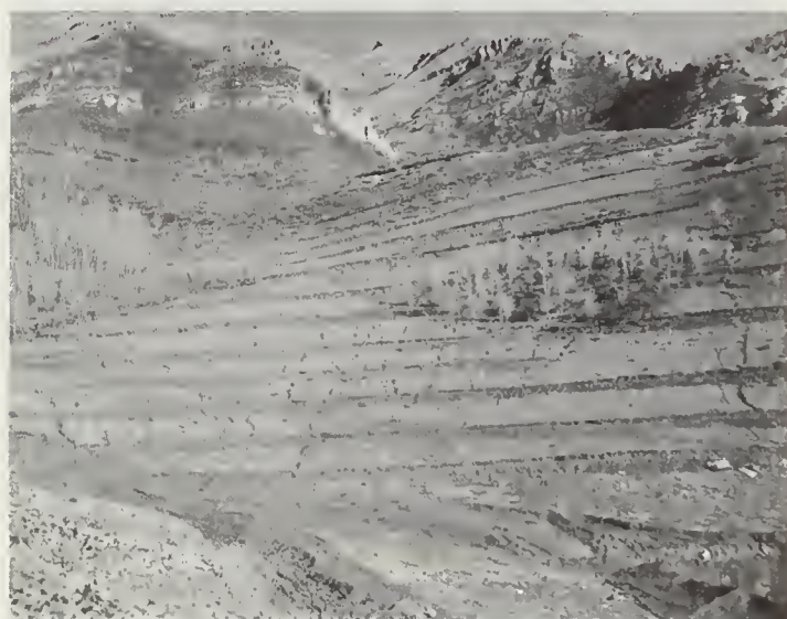
FIGURE 13. — Left, system of contour trenches constructed on Dry Creek flood-source area in fall of 1958. Trenches break up gully pattern. Right, Dry Creek area 3 years after installation of contour trench system (1961). Seeded grasses well established on soils disturbed by construction activities. Improved soil moisture condition between trenches have contributed to reestablishment of native vegetation.
