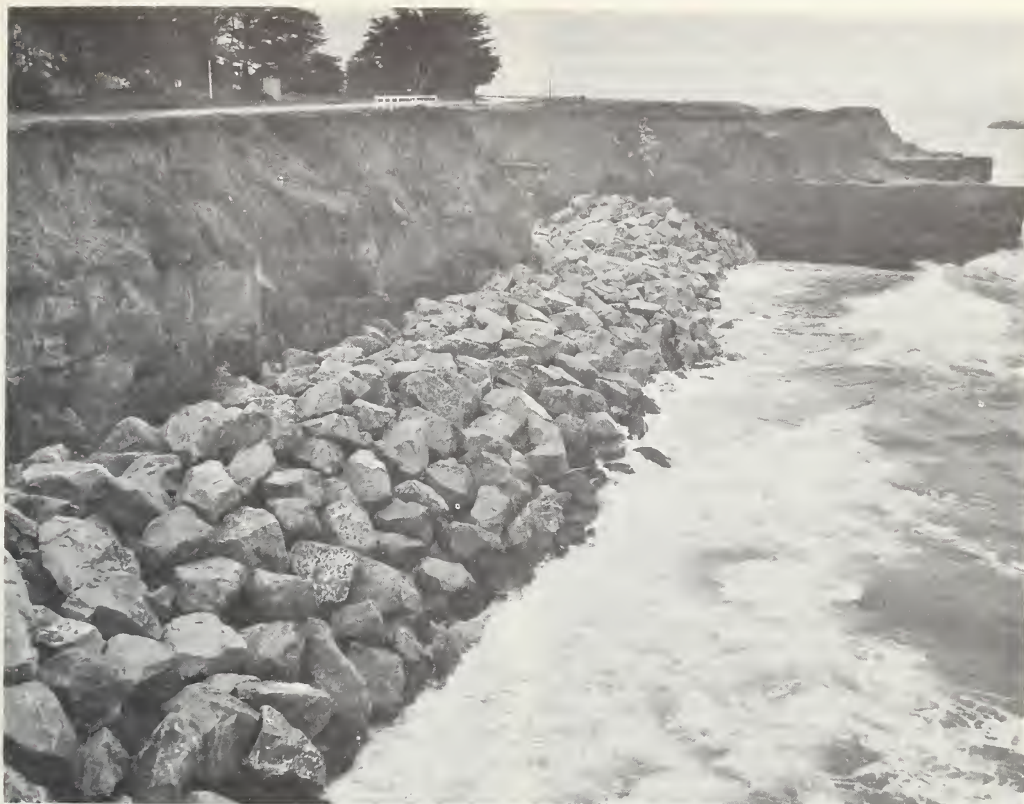
FIGURE 2. — Typical seawall unit completed in 1961.
