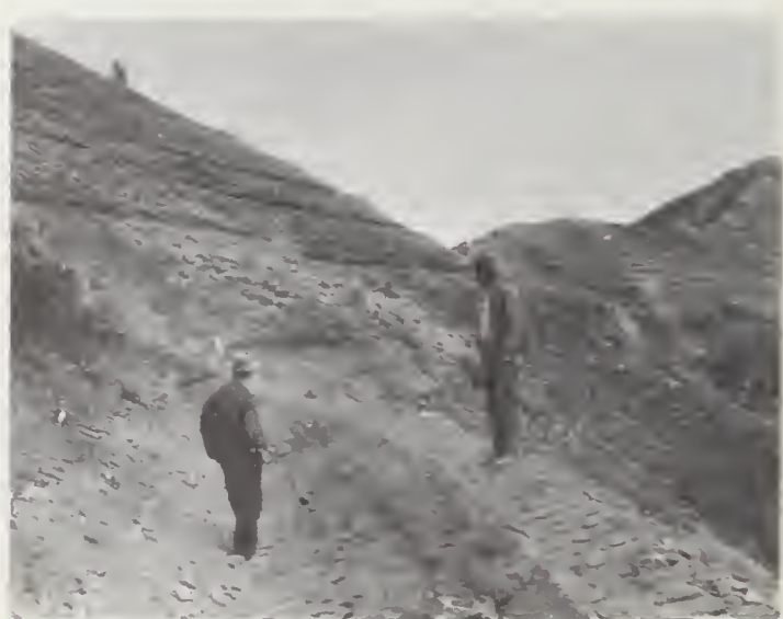
FIGURE 10. — Trench on 70-percent slope completed to standard except for cross dams or baffles, which are constructed as the tractor backs out.
