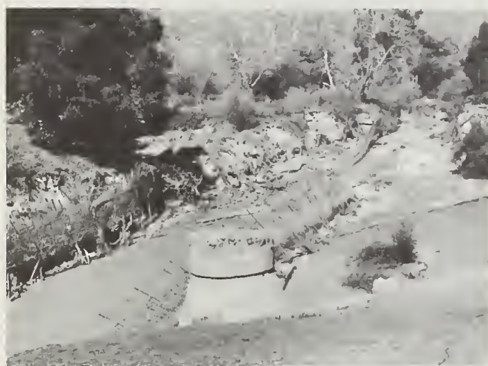
FIGURE 10. — Views showing inadequacy of pipe-and-wire fence to protect against bank erosion.
