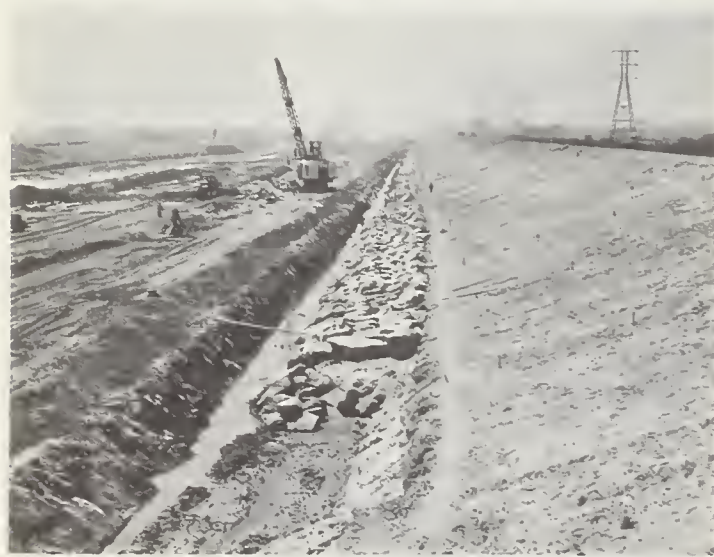
FIGURE 13. — Heavy toe stone being placed by derrick along banks of Los Angeles River channel.
