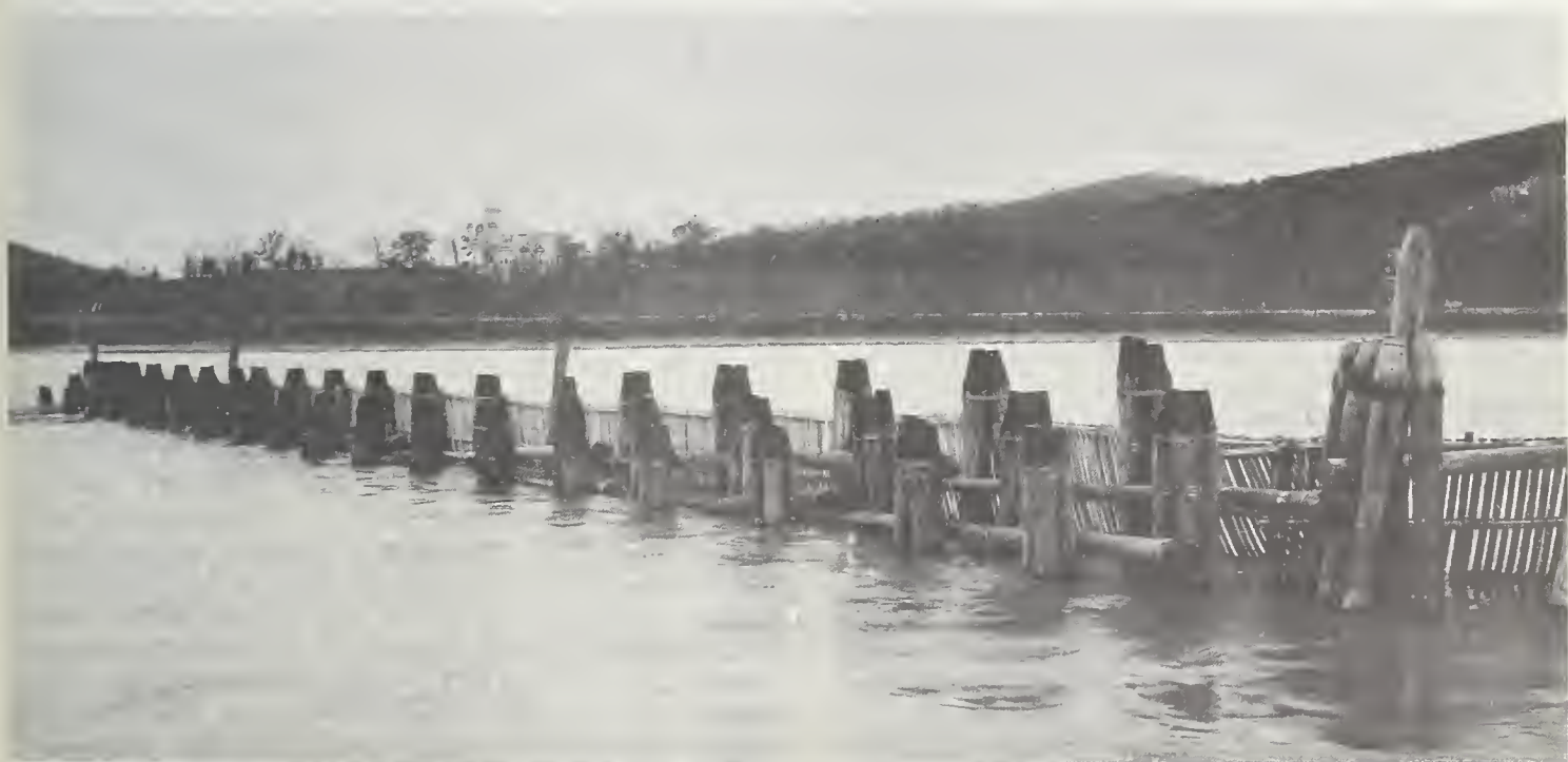
FIGURE 10. — Screen mattresses for piling dikes.
