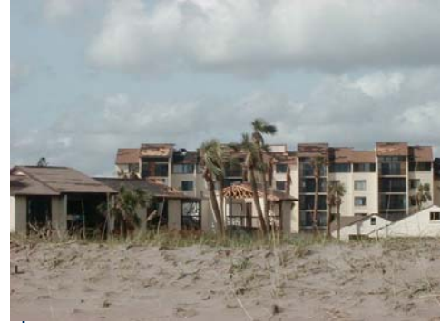
Appropriate setback regulations protect buildings and the integrity of the dune field.
