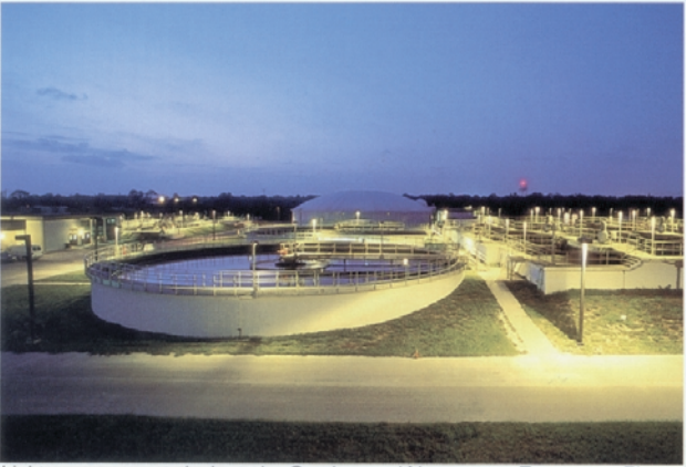
Lights come on at dusk at the South-west Wastewater Treatment Plant
