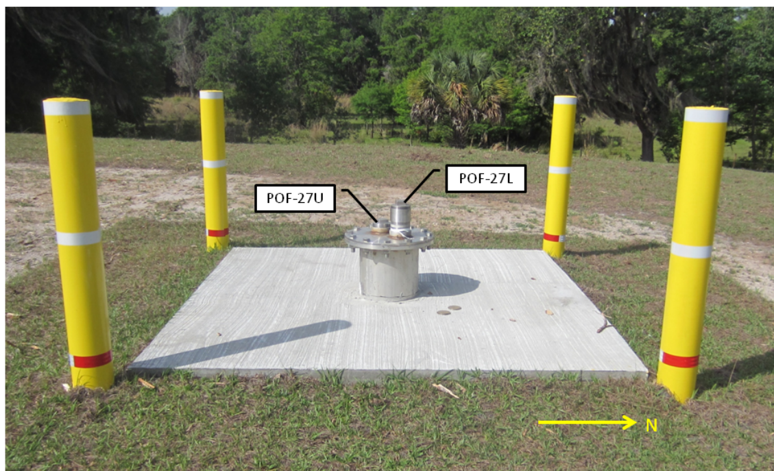
Figure 5. Final wellhead, POF-27.
