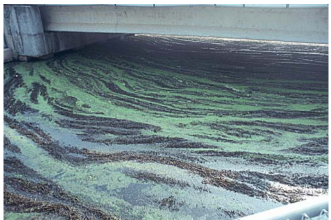
Figure 6. Hydrilla plant mass collects in front of the weir. Image taken 7/97 by Carl R. Froede Jr.
