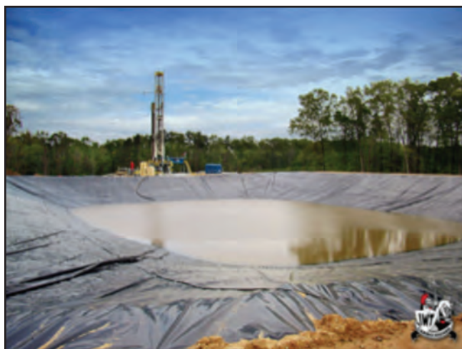
Lined pit designed to hold fluids during well drilling and completion
