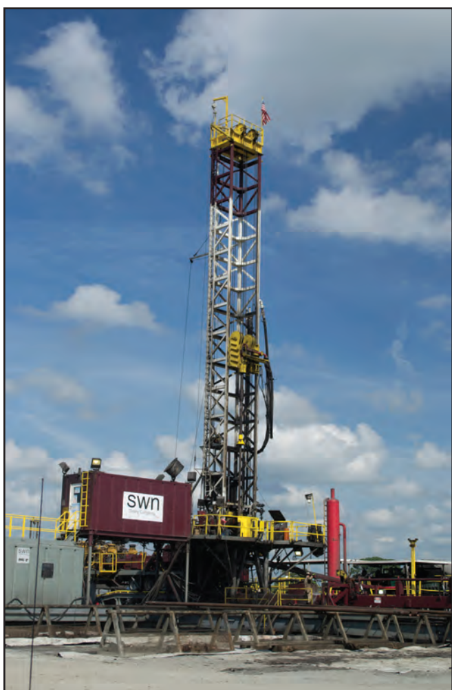
Typical rotary drilling operation
