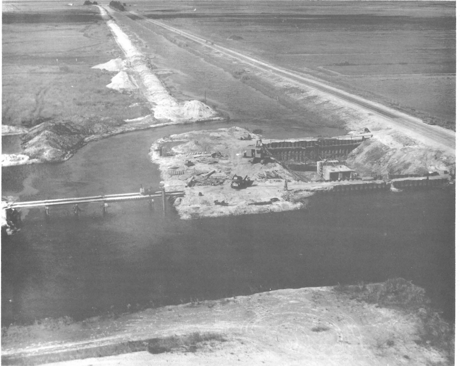
Structure S-5W, Culvert in West Palm Beach Canal near junction with Levee L-8, under construction, 14 October 1952. (Photo supplied by Flood Control District.)
