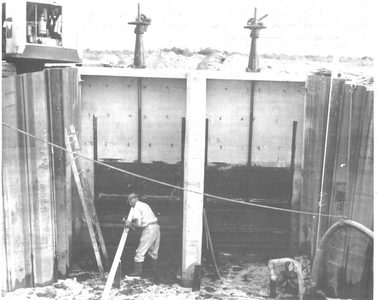
Auxiliary structure under construction by the Flood Control District in Levee L-40, for better utilization of the basic comprehensive plan. (Photo supplied by the Flood Control District.)
