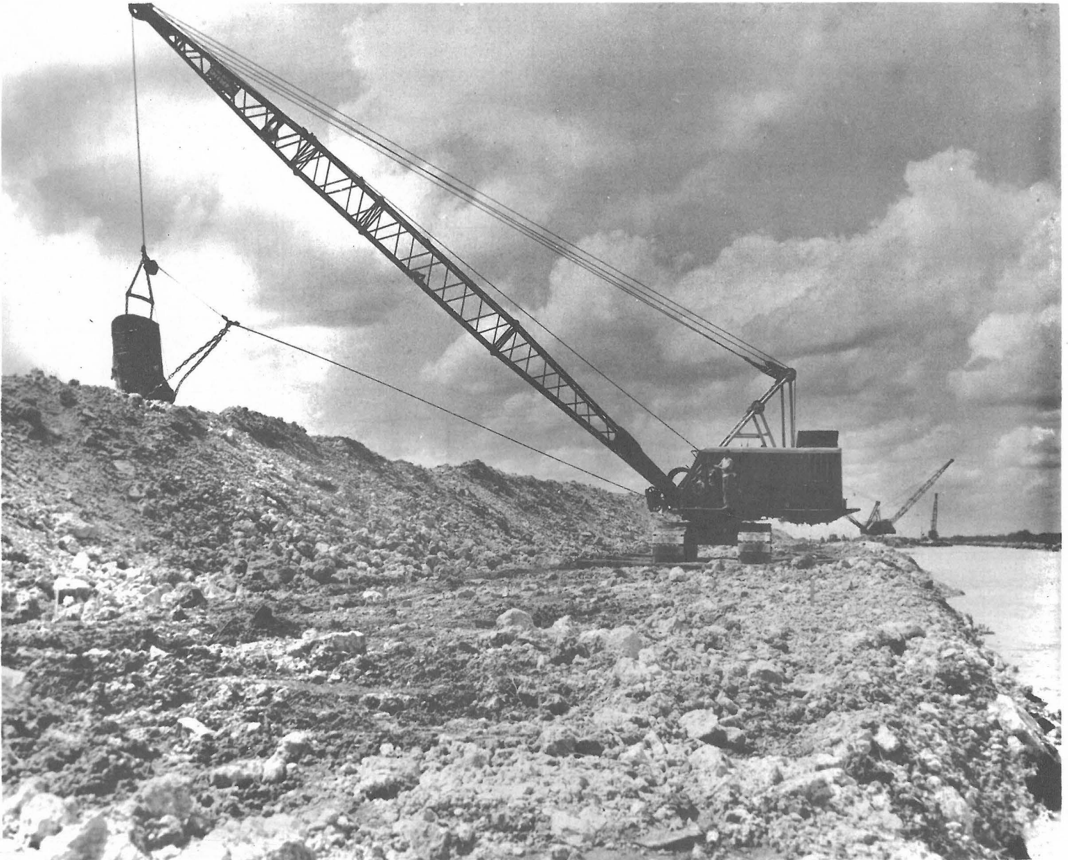
Levee L-33, Broward County, under construction, 28 April 1951. (Photo supplied by Flood Control District.)
