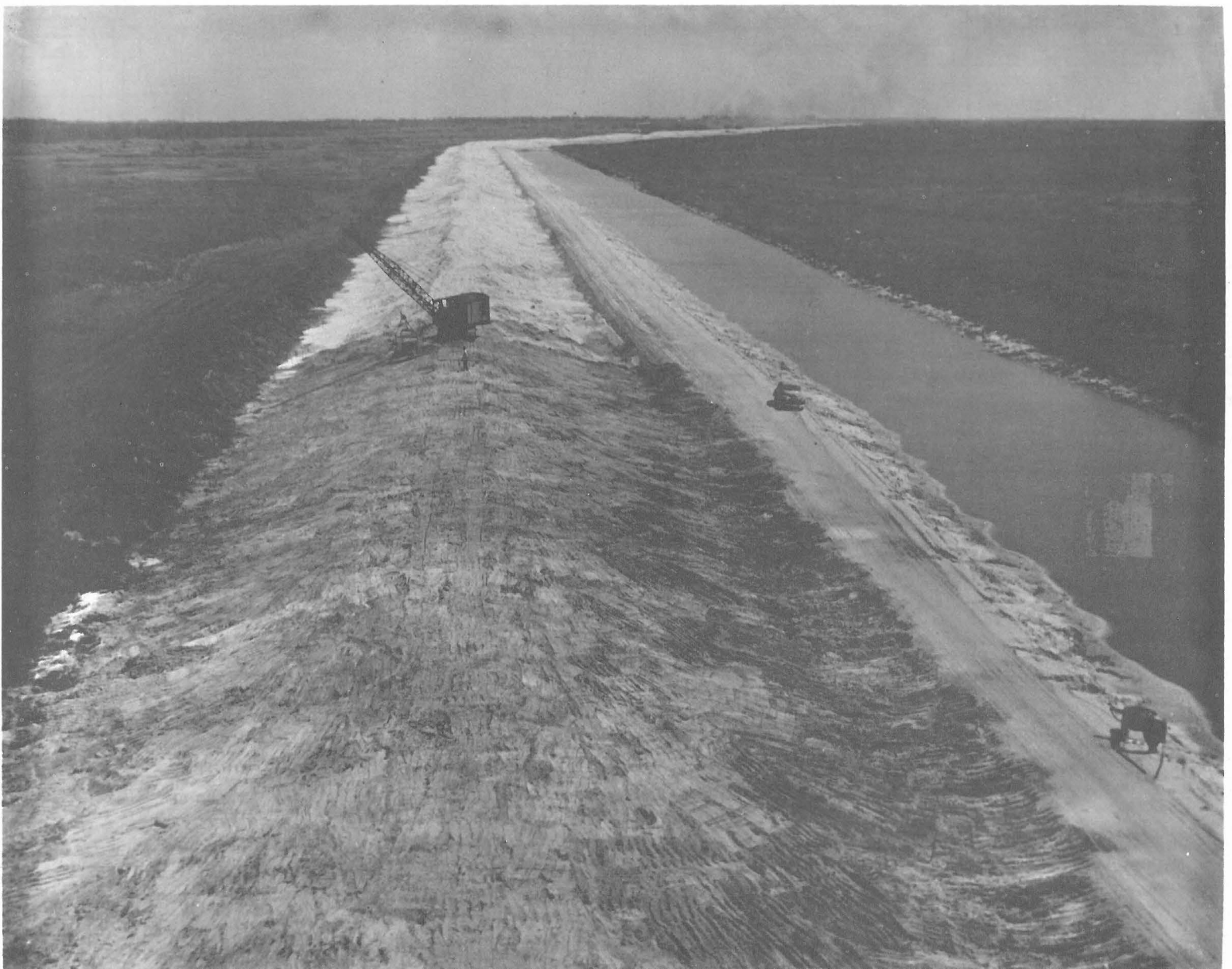
Levee L-40 in Broward County under construction. (Photo supplied by Flood Control District.)
