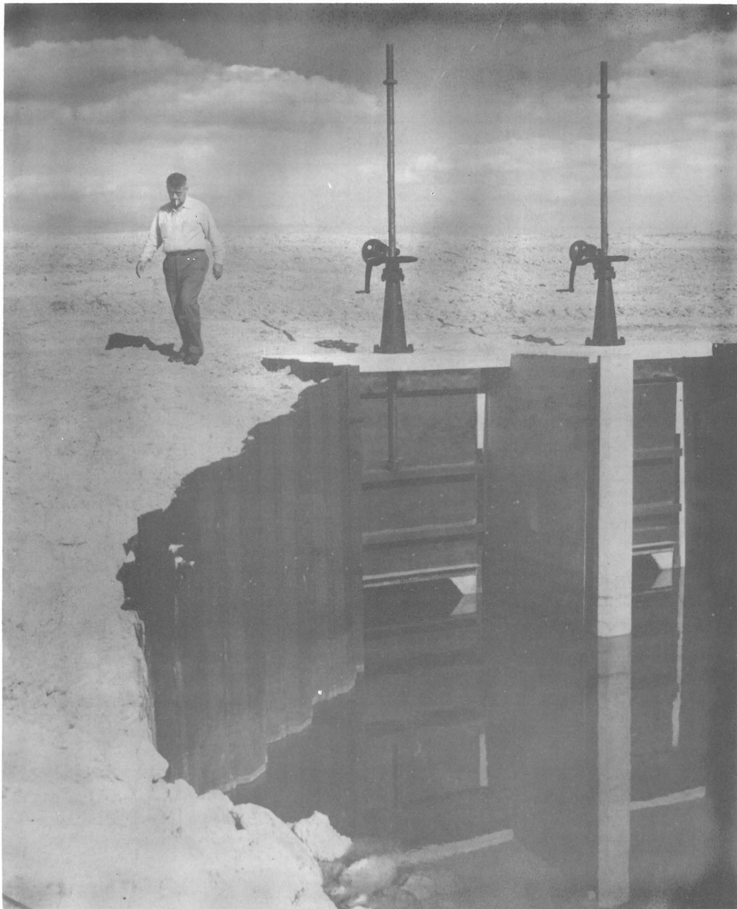
Type of auxiliary structure being constructed by the Flood Control District to better utilize the basic comprehensive plan. This structure is in Levee L-40. (Photo supplied by Flood Control District.)
