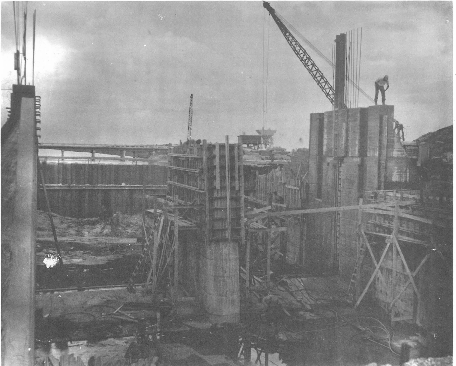
Structure S-5S, Palm Beach County, spillway at south end of Canal and Levee L-8 and north end of Conservation Area No. 1, under construction, 9 July 1953. ( Photo supplied by Flood Control District. )
