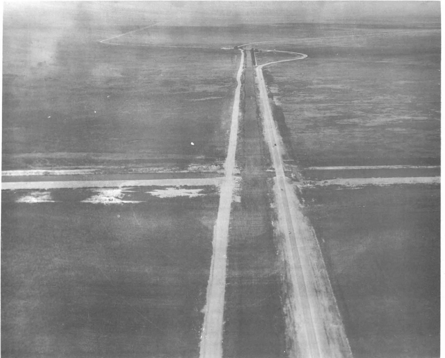
Junction of Levees L-8 and L-40 with West Palm Beach Canal, Levee L-8 to the right, 16 March 1951. (Photo supplied by Flood Control District.)
