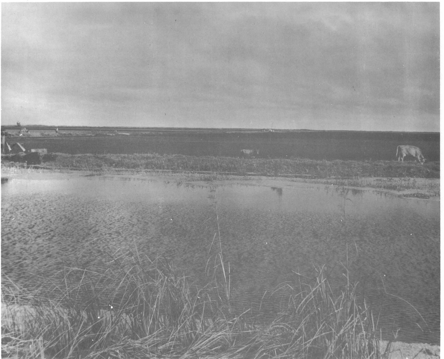
High water in Ocean Canal (Cross Canal), Palm Beach County, 23 October 1952. (Photo supplied by Flood Control District.)
