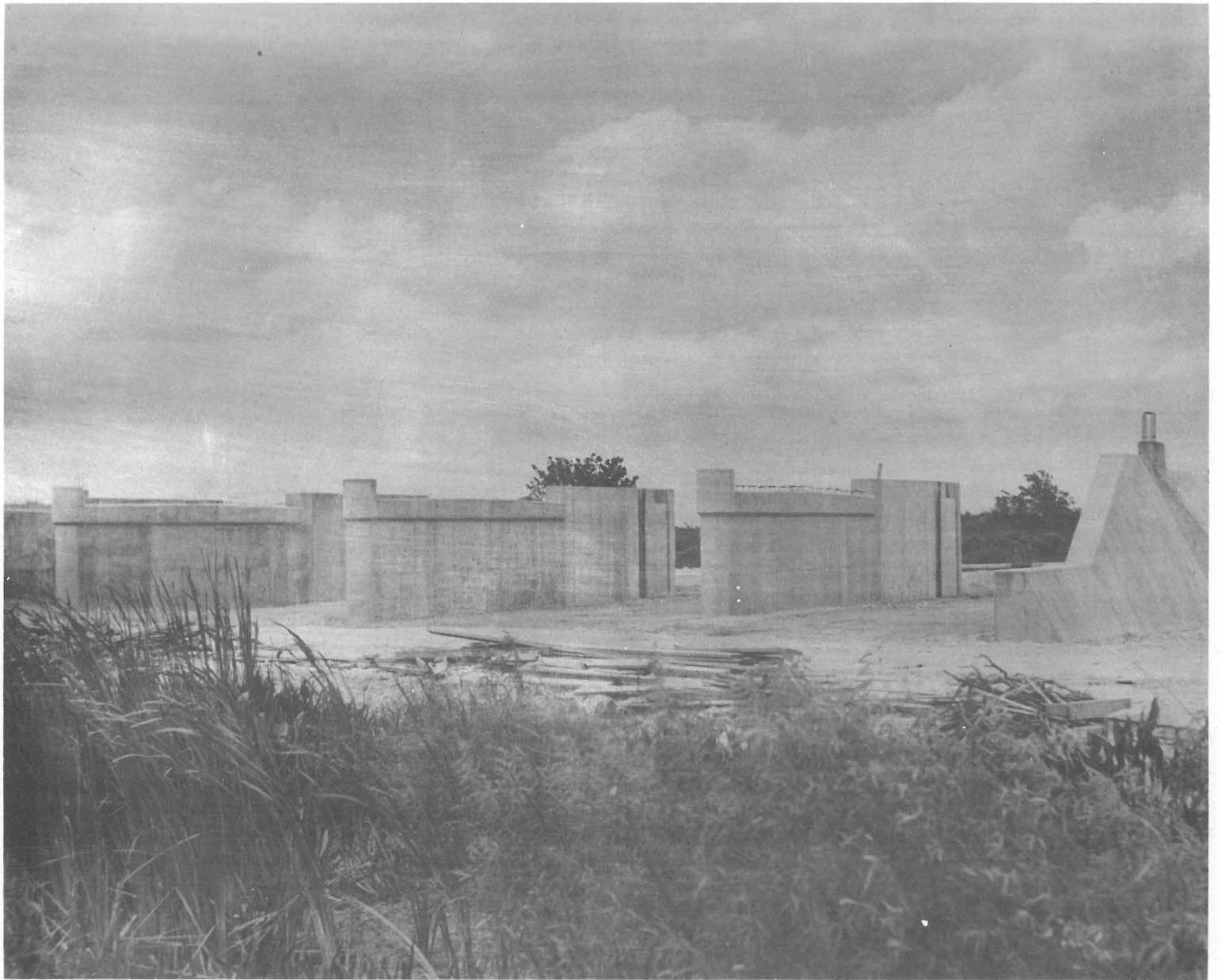
Structure S-11, (see opposite), under construction, 19 May 1953. ( Photo supplied by Flood Control District. )
