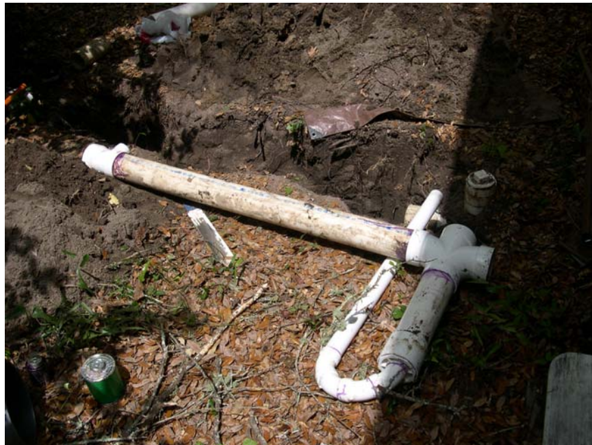
Figure 7. Plumbing for sampling raw wastewater about to be installed between the house and septic tank at site WSS-4-2. The water sensor is placed in the 4 inch opening of the 4-way PVC piece. Note the inlet clean out.
