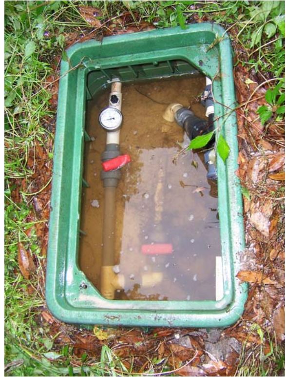
Figure 17. Pictures of site WS-4 taken on April 14, 2009. The broken plumbing evident in this picture was also reported in September 2008. The broken pipe causes the effluent to fill the control box instead of going to the drain field.
