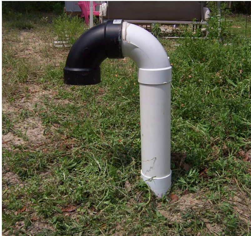
Figure 16. Picture taken on 04/14/09 of a vent pipe typical of FAST installations. Note the coupler at ground level. In order to take a sample, the pipe was cut and repaired with the coupler. The black piece is a charcoal filter installed due to odor complaints. This site is in a high density neighborhood with 10 PBTS in a 1.25-acre area, which are apparently creating an odor problem.
