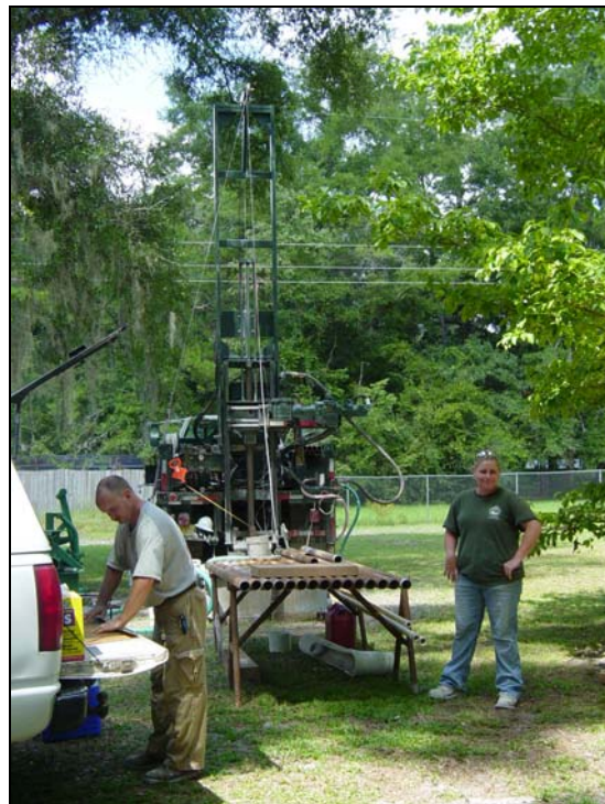
Figure 1.4.4: FGS drilling the well (Brie Coane and Ken Campbell)
