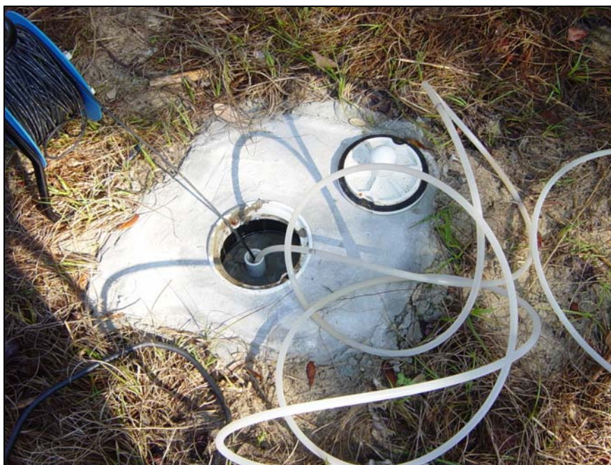
Figure 1.1.12: WRB background monitoring well number 2.
