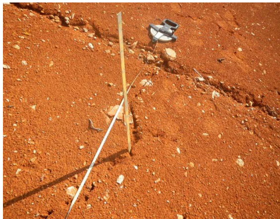
Figure 7. The clay liner shown here is the sole confining entity separating the hog waste in the lagoons from the underlying Boone Formation. This photo, taken after construction of the liner, indicates that it has numerous chert fragments up to fist size within the clay, and desiccation cracks, and that erosion rills have eroded some of the thickness. These features reduce its ability to confine. The liner was required to be 30 cm thick, but the owners of the CAFO increased that to 45 cm. Photo courtesy of Tony Morris (ADEQ).
