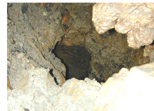
One of the small conduits draining the lower sink cavity.
