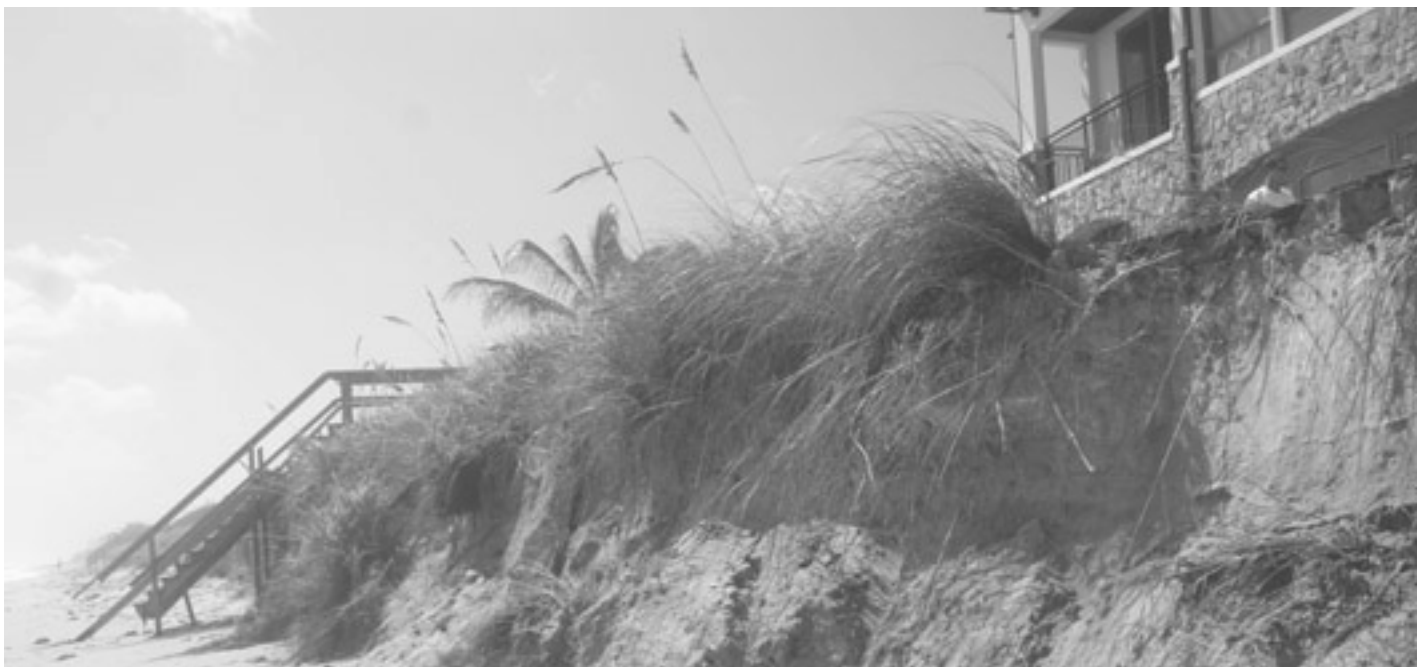
An Example of Beach Erosion and its Effects from South Brevard County.
