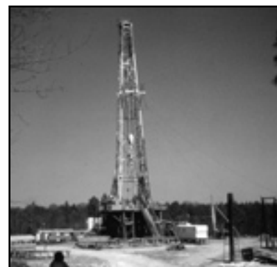
Typical 1970's era heavy duty drill rig in Northwest Florida. Capable of reaching petroleum deposits in the Smackover Formation at depths of 3 miles.
