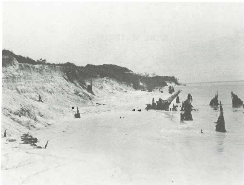
Figure 10. St. Andrews State Recreation Area. View north along the west side of the Land's End Canal. The tree stumps in the water and the step scarp are signs of active erosion.
