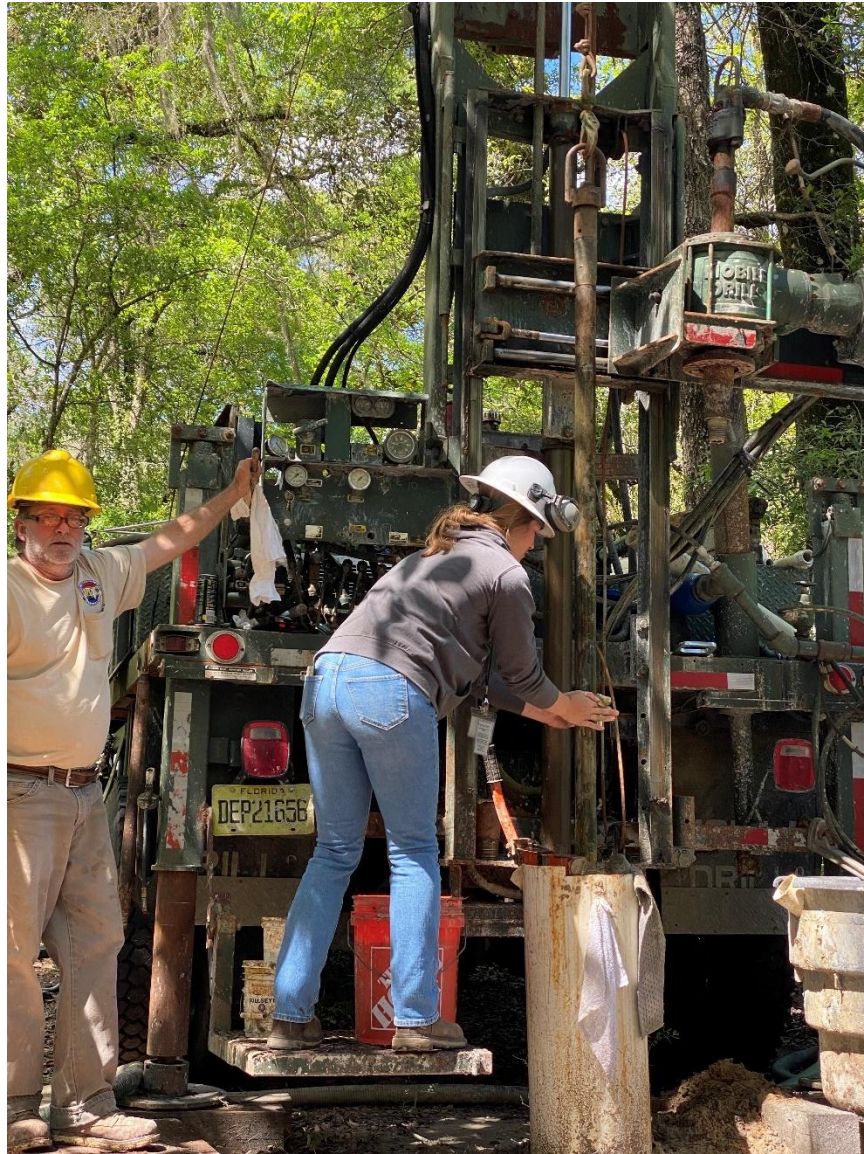
Figure 6. FGS staff geologists and drilling specialists recover DPT rod at a site being converted to rotary methods. Surficial unconsolidated sand and clay beds, when saturated, proved difficult for DPT penetration. Swelling clays at this site locked the DPT outer rods downhole at depth. The Mobile Drill B31 was outfitted with a modified coupling to recover DPT rods and sample.
