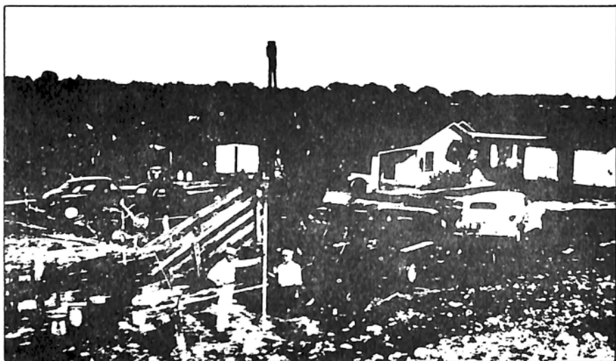
A. DRILLING WELL G 513
