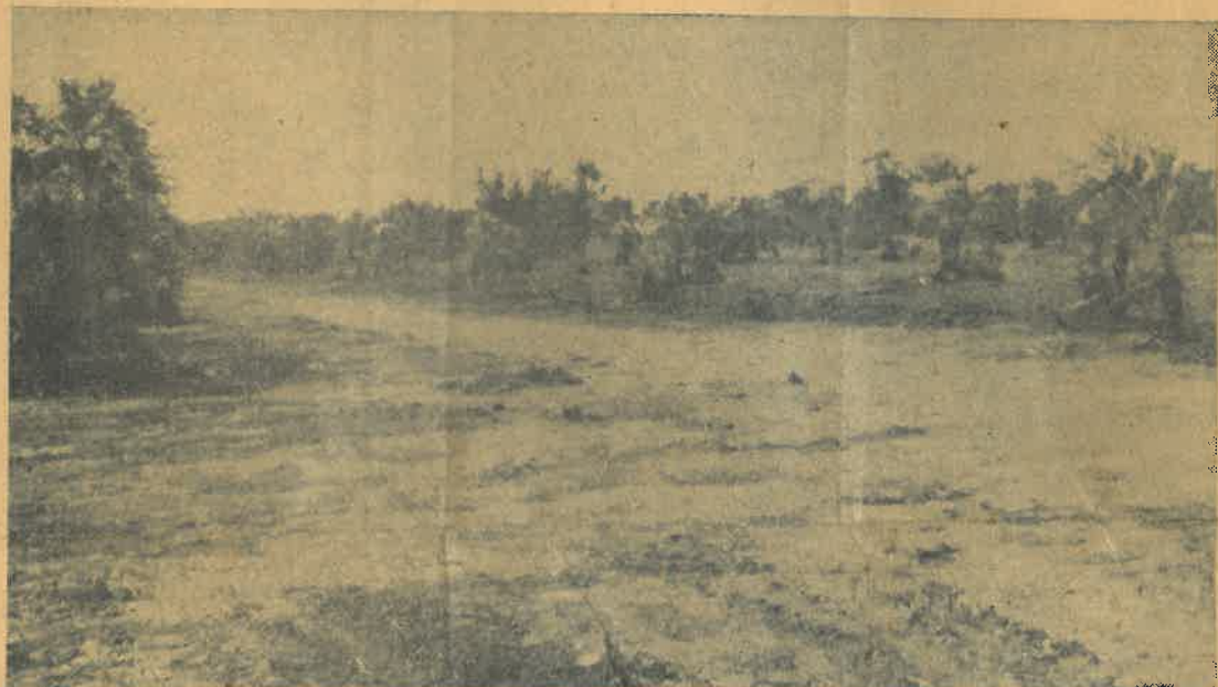
CEMETERY SITE —First unit of new cemetery on Big Coppitt Key is on its way to completion on this 11-acre tract. The builders, Southern Keys Cemetery Corporation, say the site will be completed in several weeks. Plans also call for the first unit of a mausoleum to be built there.
