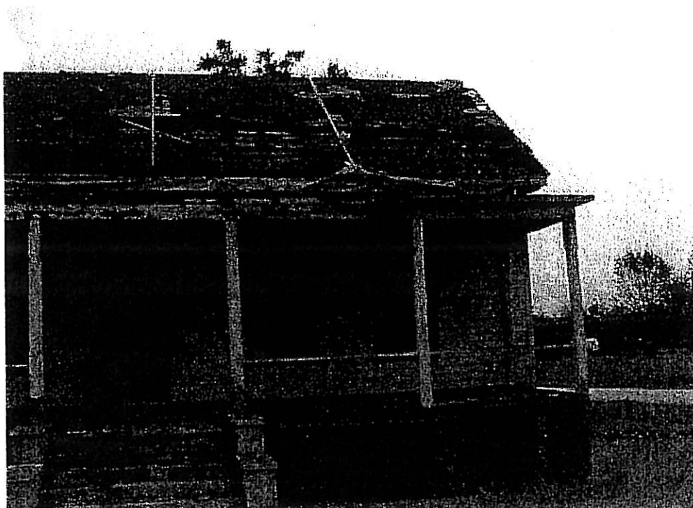
Photo #2 – Front Porch, Damage Roof, South Elevation
