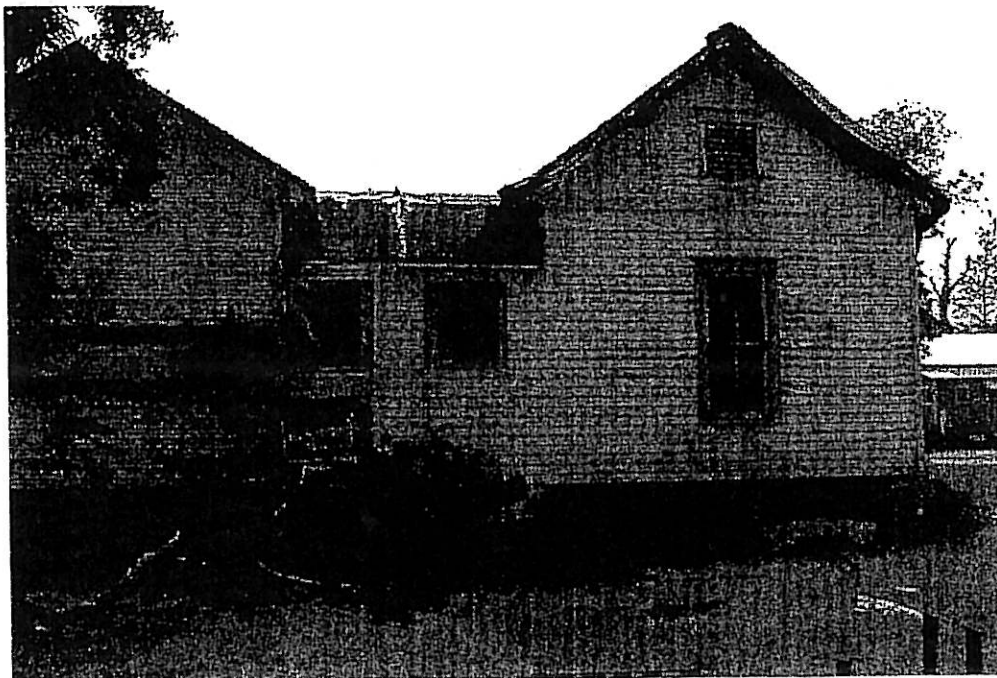
Photo #7 – North Elevation – Flat Roof over Original Porch
