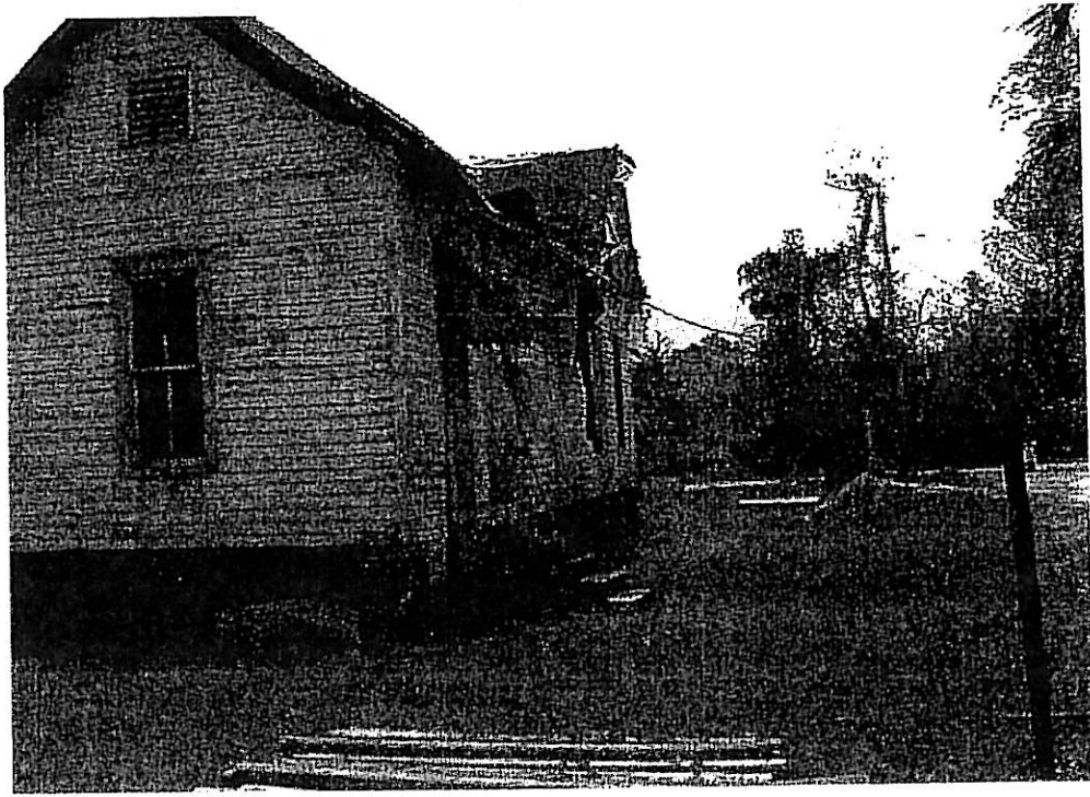
Photo #8 – North West Corner Looking South
