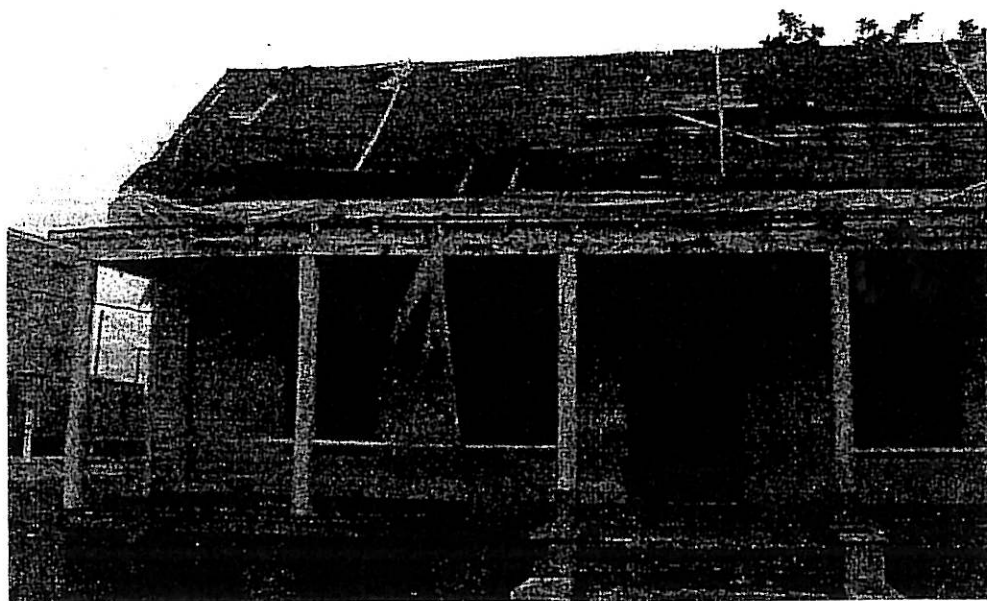
Photo #1 – Front Porch, Damaged Roof – South Elevation
