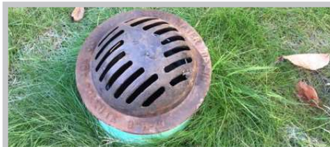
Beehive Overflow Filter Riser for collection of gross solids during major storm events
