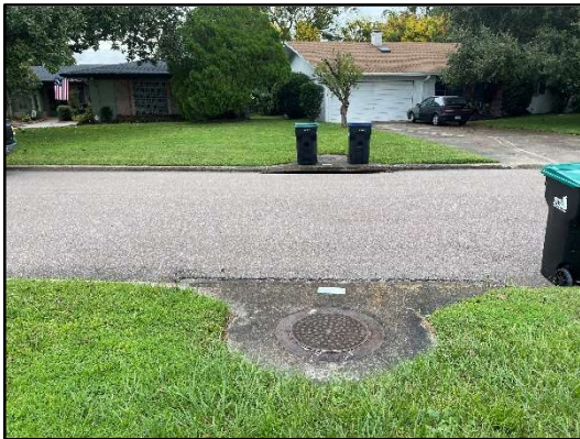
4006, curb inlets on Bass Lake Blvd. looking west toward Bass Lake outfall BLA4
