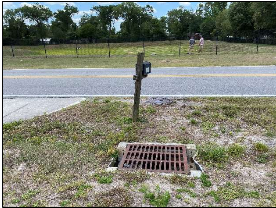
2361, grated drop inlet on north side of Grant St. looking south to retention pond
