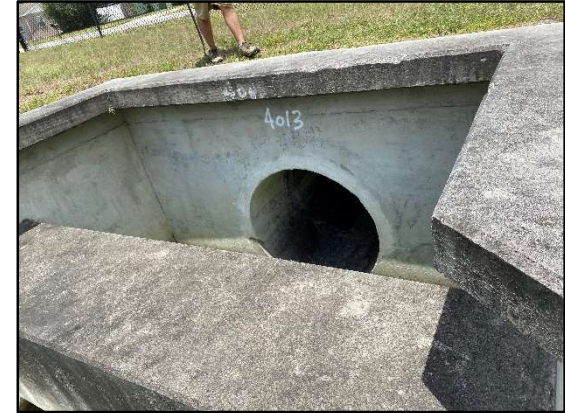
2365, culvert headwall in retention pond looking north toward Grant St.
