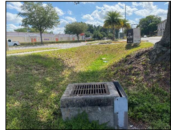
2324, overflow weir in retention pond on south side of Michigan St., looking east
