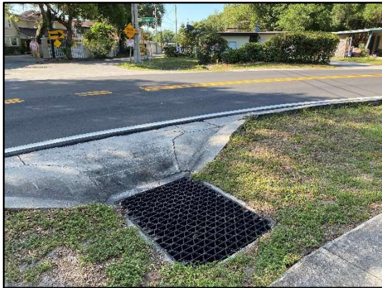
2298, grated drop inlet from Crystal Lake Dr. to outfall BLA1, looking south
