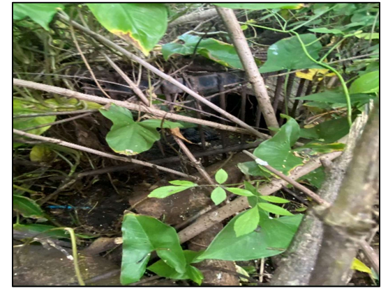
2398, barred culvert headwall at outfall BLA 2, looking northeast toward Jersey Ave.
