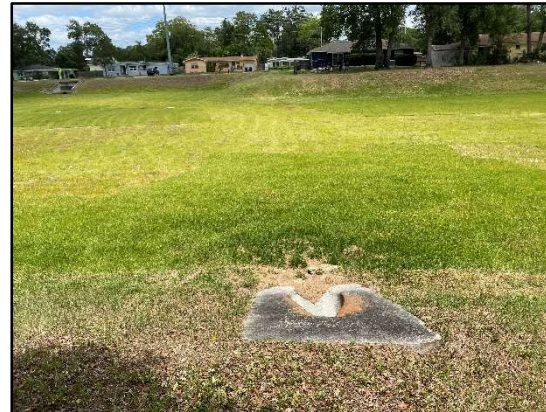
2371, mitered end section at south end of retention pond, looking north toward Grant St.
