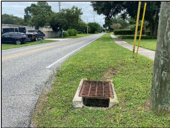
4004, grated drop inlet on the south side of Raeford Rd., east of Peel Ave. looking east
