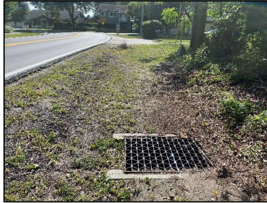
2308, grated drop inlet on south side of Crystal Lake Dr. to outfall BLA1, looking east
