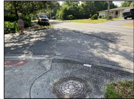
2310, curb inlet at Lassek Dr. and Crystal Lake Dr. looking east
