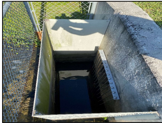
2290, interior of outfall overflow weir at BLA1
