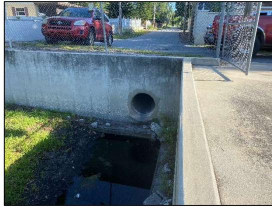
2279, drainage pipe from Crystal Lake Dr. to retention pond BLA1, looking north
