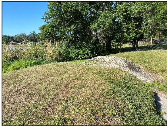
2281, riprap swale into Bass Lake from retention pond at BLA1, looking southeast
