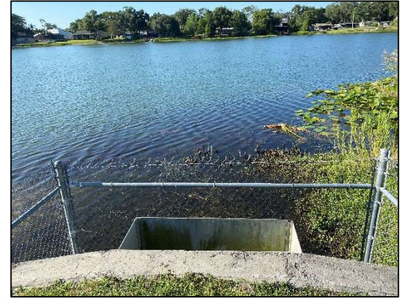
2285, overflow weir and outfall at BLA1, looking south
