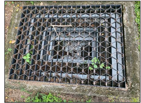
4003, debris strainer in each grated drop inlet along the north side of Raeford Rd.
