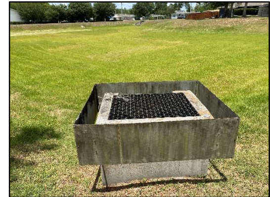
2372, grated drop inlet overflow weir in retention pond, looking northwest
