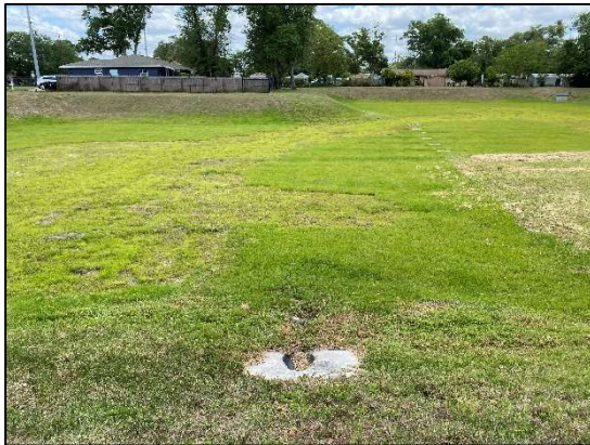
2368, mitered end section at west end of retention pond, looking east toward Rest Haven Ave.
