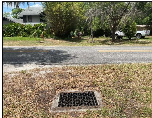
2388, grated drop inlet on south side of Raeford Rd. looking north toward BLA3
