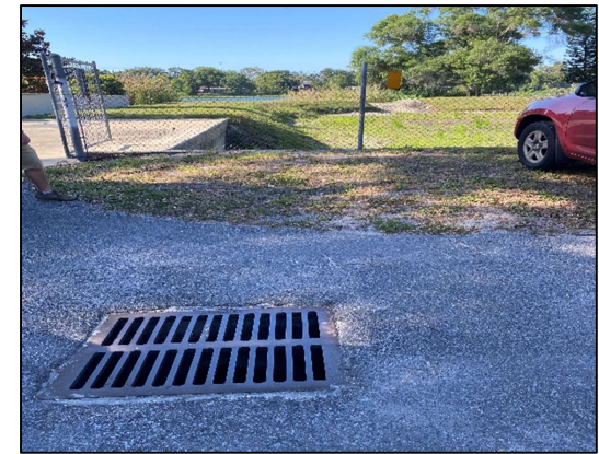
2291, grated drop inlet to outfall at BLA1, looking south
