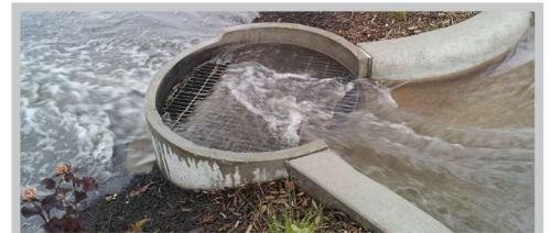
Rain Guardian Turret for curbline pretreatment and energy dissipation
