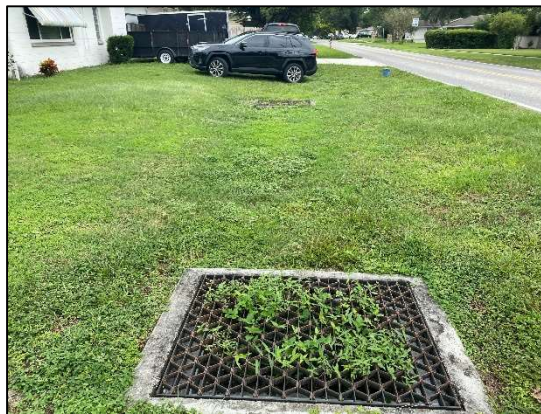
4005, 2 grated drop inlets on the north side of Raeford Rd., east of Peel Ave. looking east
