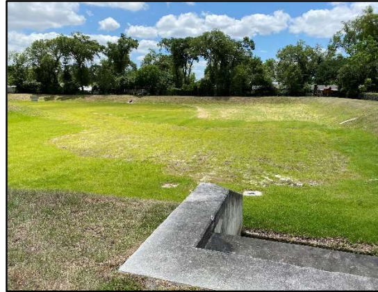
2366, culvert headwall in retention pond looking south from Grant St.
