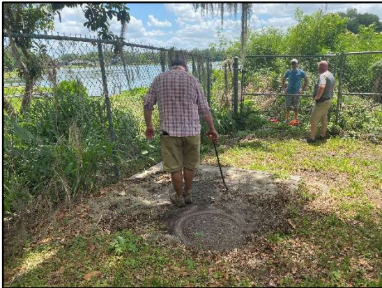
2396, manhole at outfall BLA2, looking southwest toward Bass Lake
