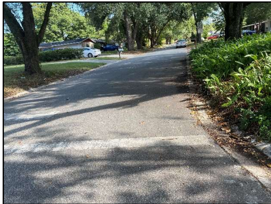
2312, concrete flowlines and slope on Lassek Dr. toward Crystal Lake Dr., looking north
