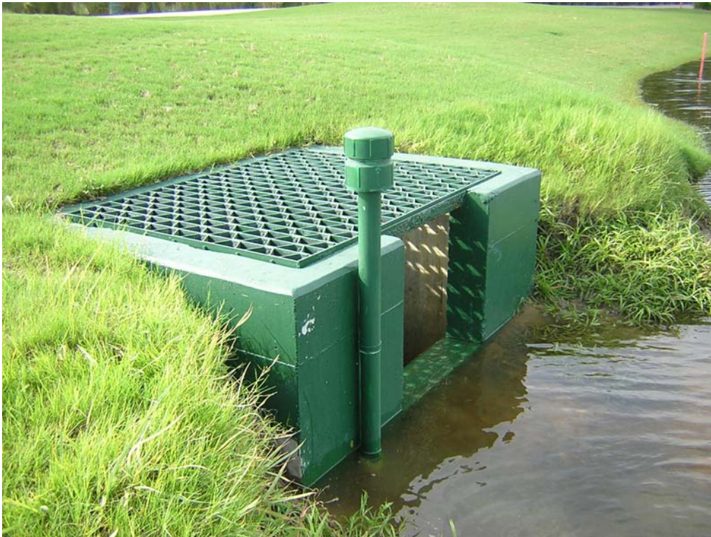
Shadow Wood Preserve L8 outfall 7-18-08 showing high water conditions and piezometer.
