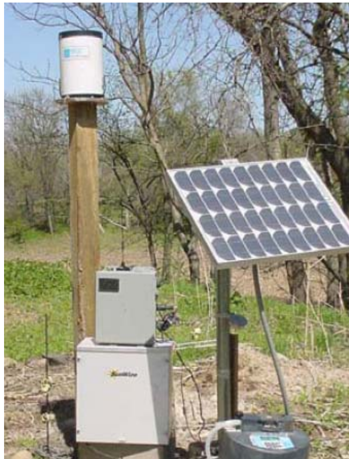
Figure 3: ISCO Series 674 Rain Gauge and Solar Panel
