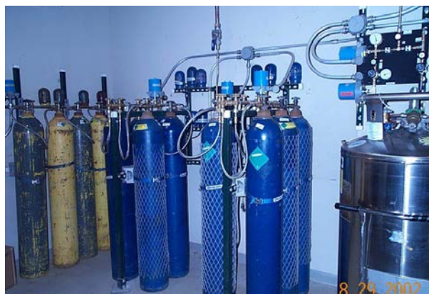
Figure 11.3 Typical Compressed Gas Manifold
