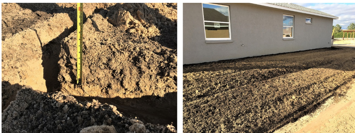
Figure 3. Check for a general 6-inch incorporation depth, 4-inch minimum in small areas and level the amended surface after compost incorporation. Credit: UF/PREC.
