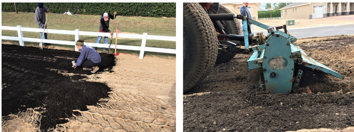
Figure 2. Hand repair any unevenly applied areas and incorporate compost using a rototiller. Credit: UF/PREC.
