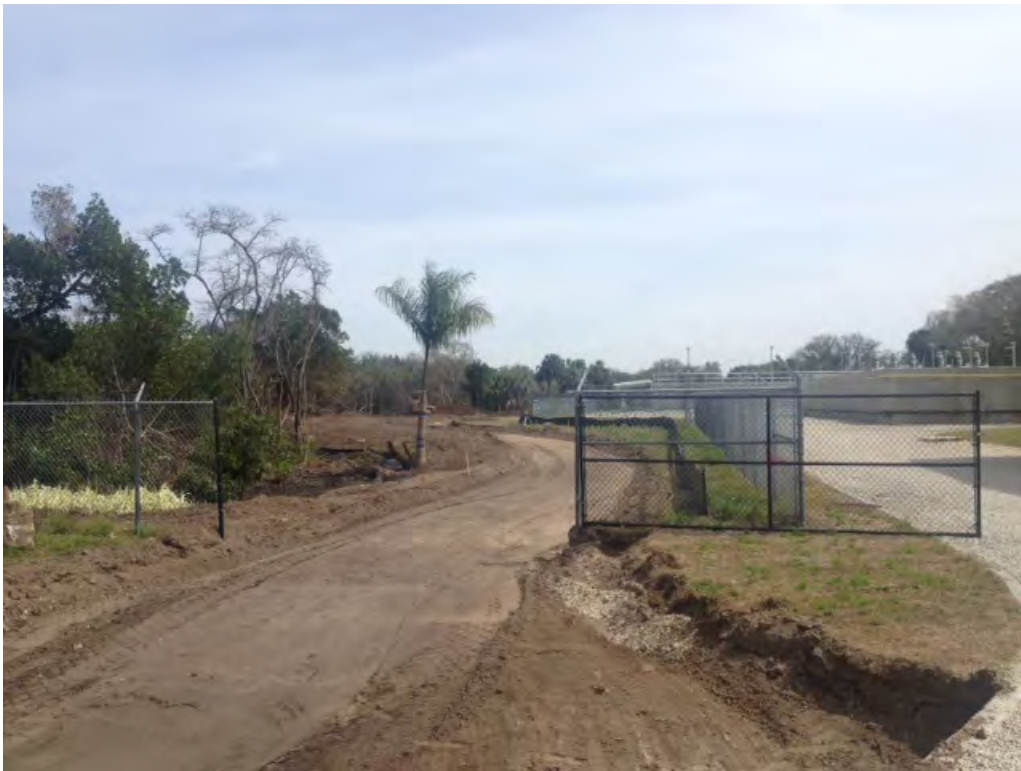
FIGURE B-6: CITY OF FORT MYERS FORD STREET FILTER MARSH CONSTRUCTION
