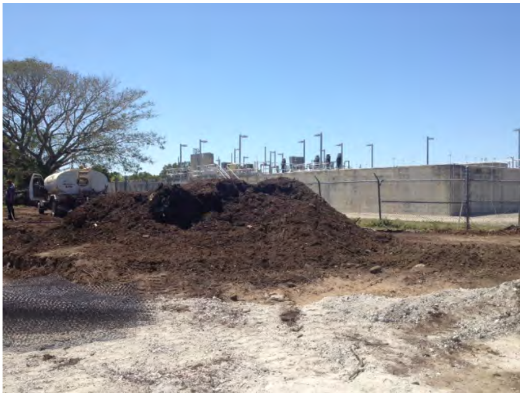
FIGURE B-4: CITY OF FORT MYERS FORD STREET FILTER MARSH CONSTRUCTION
