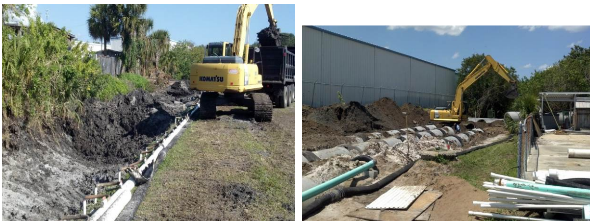
FIGURE 7: CITY OF CAPE CANAVERAL CENTRAL DRAINAGE DITCH PROJECT CONSTRUCTION
