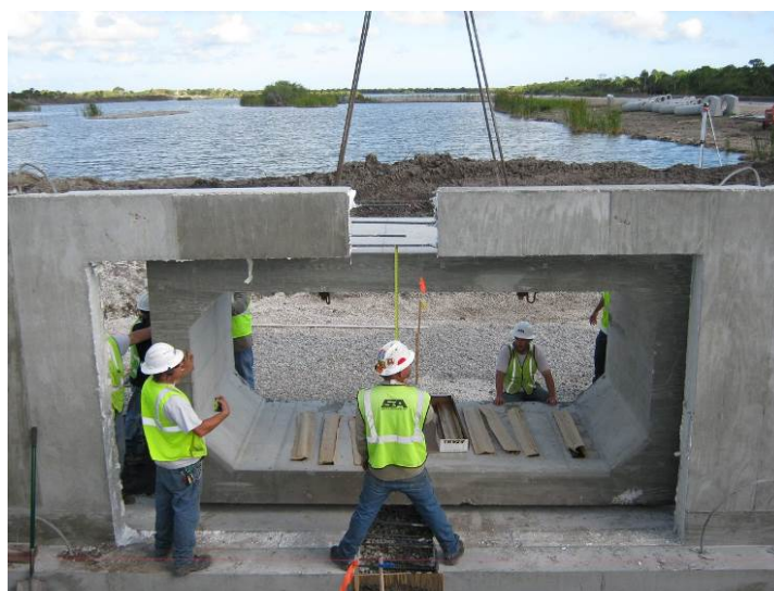
FIGURE 3: BREVARD COUNTY PINE ISLAND PROJECT UNDER CONSTRUCTION
