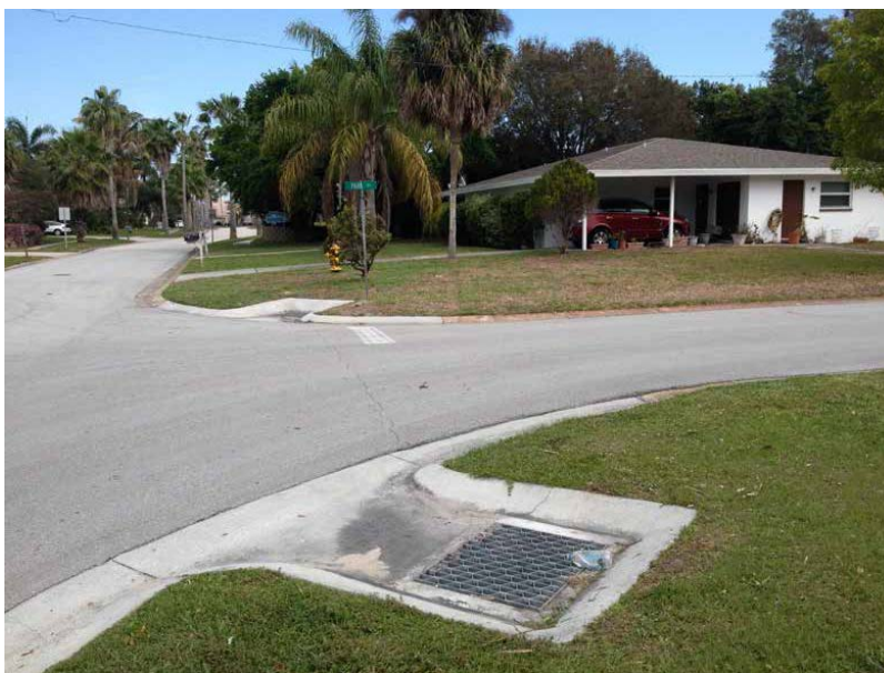
FIGURE 14: CITY OF INDIAN HARBOUR BEACH PARK STREET INLET AND EXFILTRATION TRENCH
