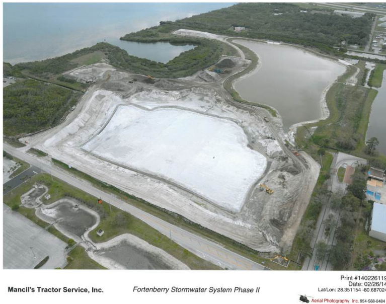
FIGURE 6: BREVARD COUNTY FORTENBERRY POND UNDER CONSTRUCTION
