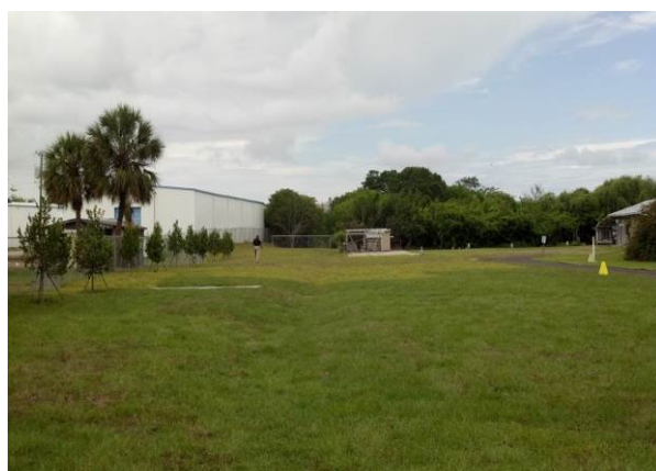
FIGURE 8: CITY OF CAPE CANAVERAL COMPLETED CENTRAL DRAINAGE DITCH PROJECT
