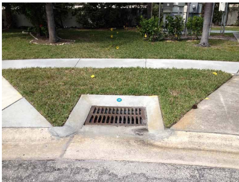
FIGURE 16: CITY OF INDIAN HARBOUR BEACH INLET AT HAWTHORNE COURT WEST AS PART OF THE LIME BAY EXFILTRATION PROJECT
