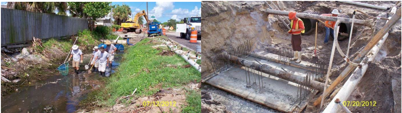
FIGURE 17: CITY OF SATELLITE BEACH CASSIA PHASE III PROJECT UNDER CONSTRUCTION
