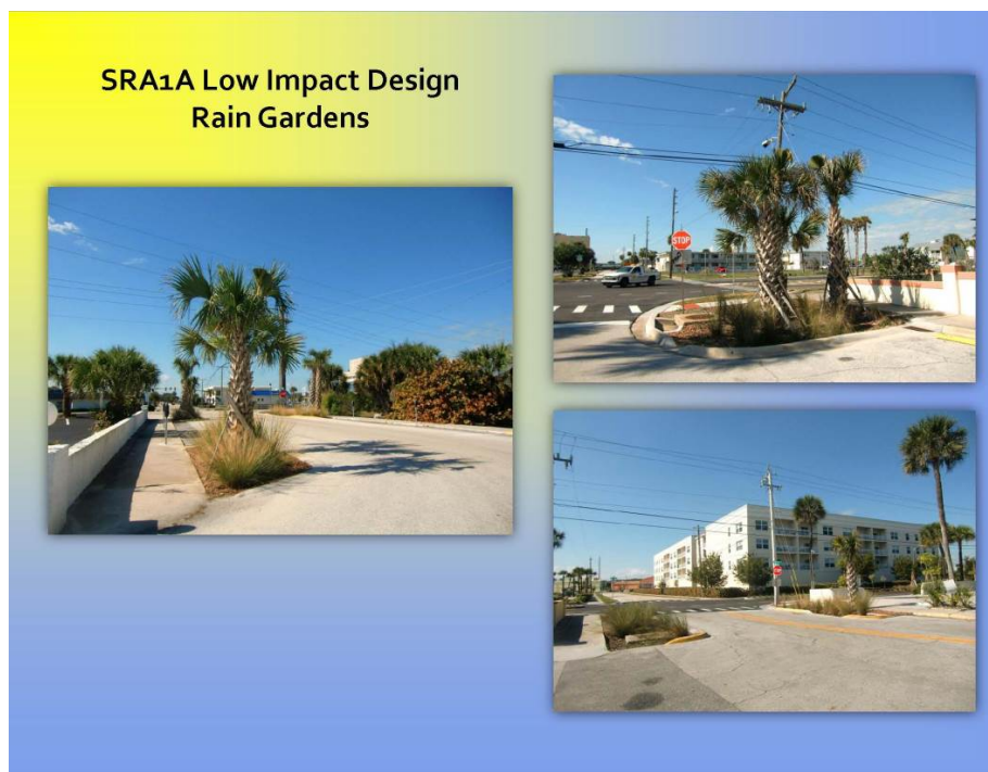
FIGURE 12: CITY OF COCOA BEACH STATE ROAD A1A BIOSWALES PROJECT
