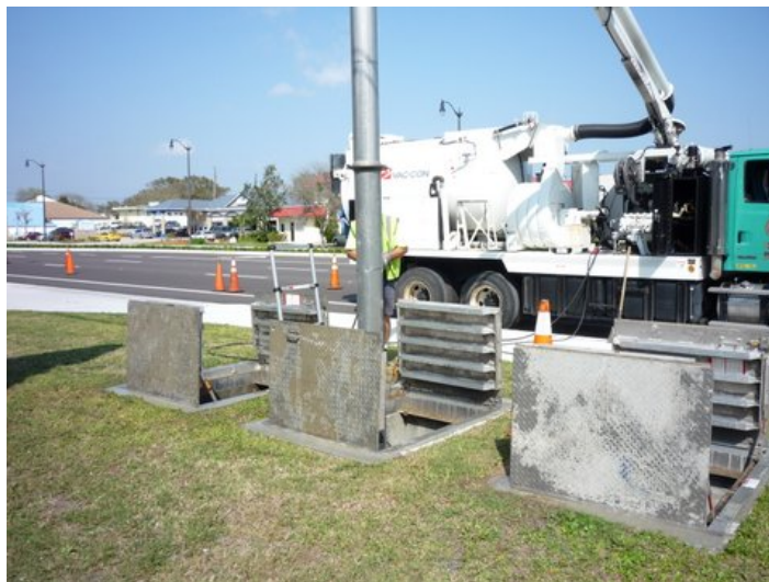
FIGURE 11: CITY OF ROCKLEDGE BAFFLE BOX CLEAN OUT
