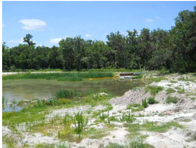
SOLARY CANAL PROJECT
