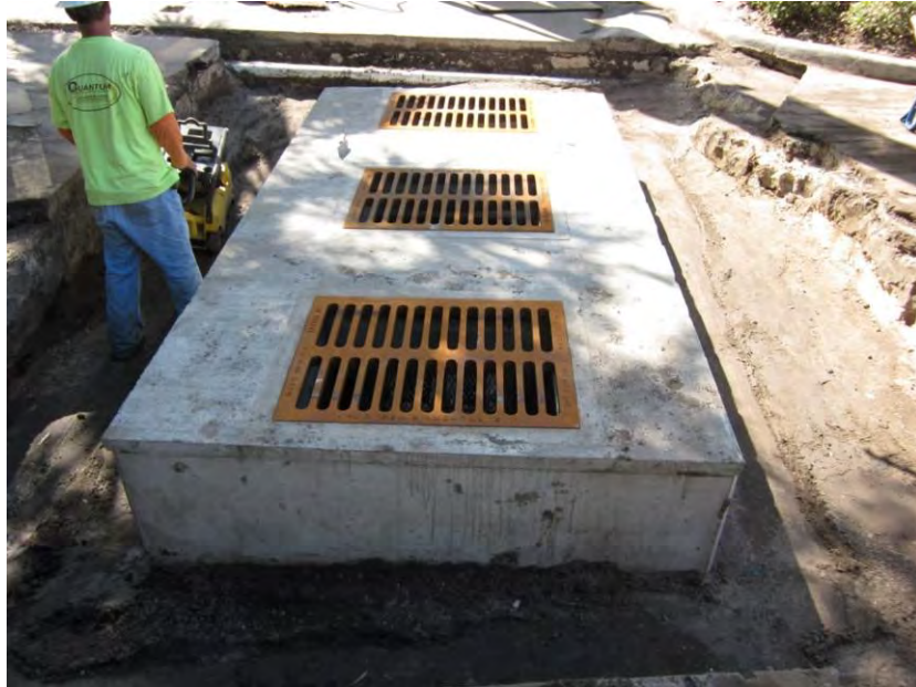
INSTALLATION OF THE PACKWOOD AVENUE BAFFLE BOX
