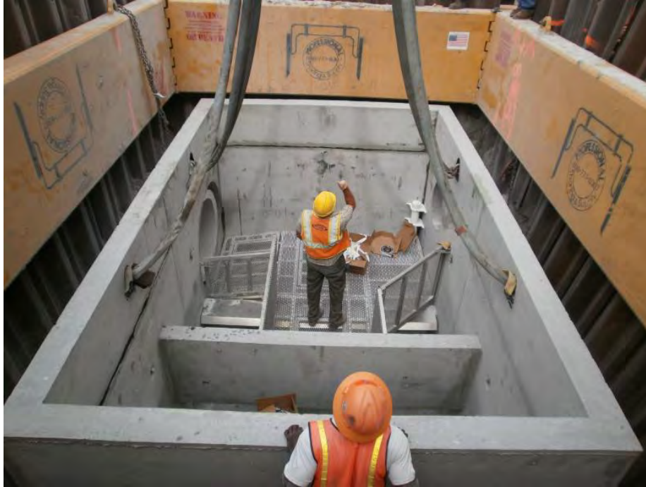
FIGURE 4: CITY OF CASSELBERRY INSTALLATION OF A BAFFLE BOX WITH MEDIA FILTRATION TO PROTECT GEE CREEK
