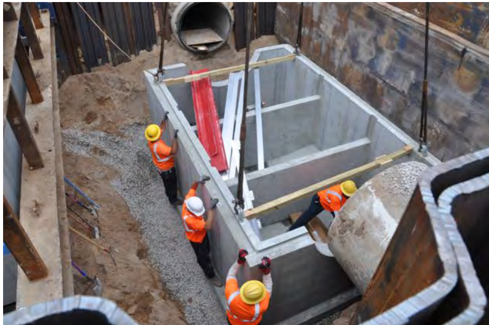
INSTALLATION OF A BAFFLE BOX AT MORSE BOULEVARD
