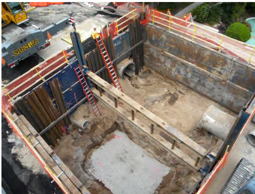
FIGURE 9: CITY OF WINTER PARK INSTALLATION OF TWO 2 ND GENERATION BAFFLE BOXES AT MORSE BOULEVARD
