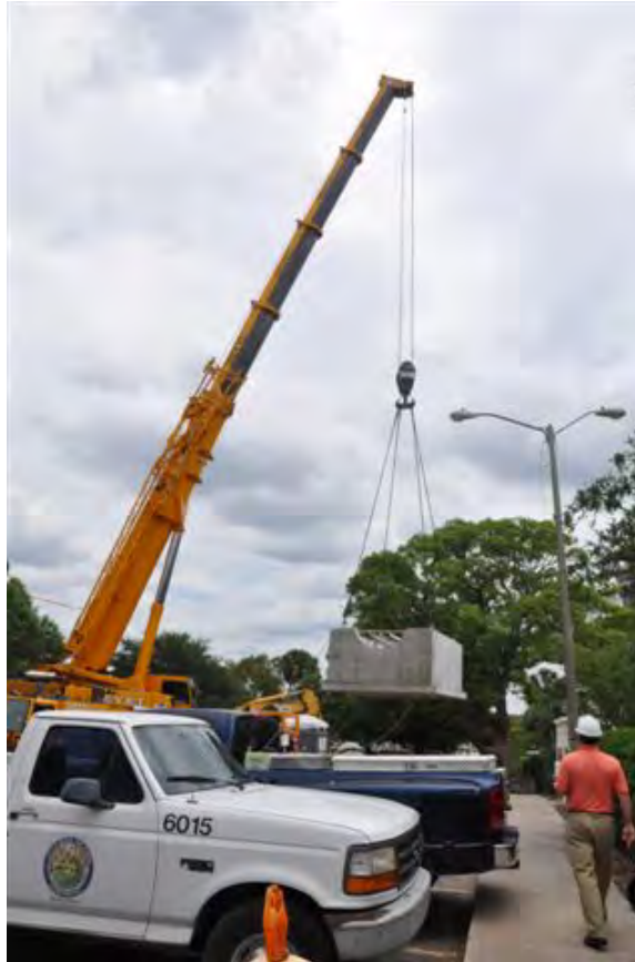
INSTALLATION OF A BAFFLE BOX AT MORSE BOULEVARD
