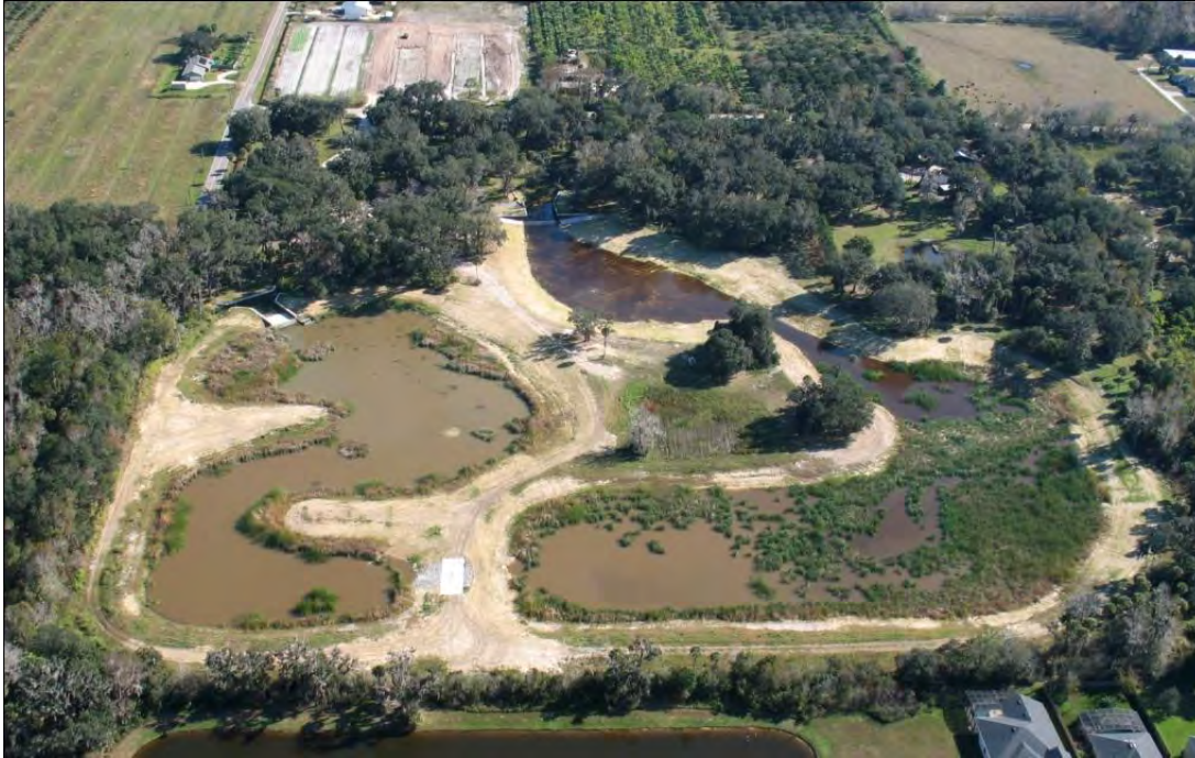
FIGURE 10: AERIAL IMAGE OF THE SOLARY CANAL STORMWATER TREATMENT AREA
