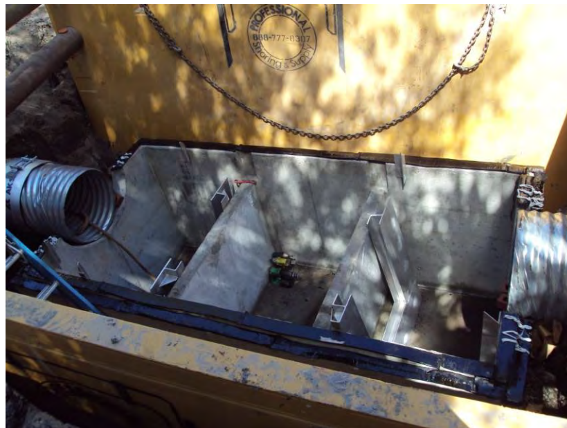
FIGURE 6: CITY OF MAITLAND PACKWOOD AVENUE BAFFLE BOX INSTALLATION
