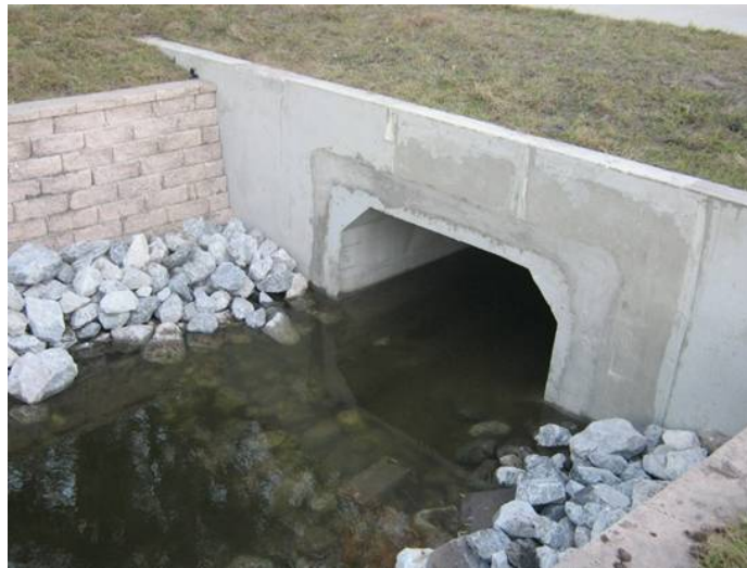
FIGURE 6: CITY OF LONGWOOD FAIRY LAKE OUTFALL COMPLETED
