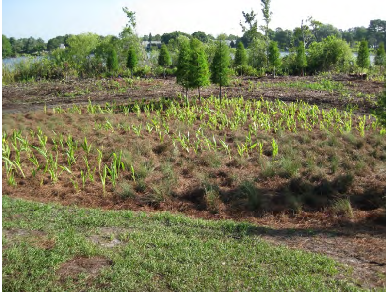
FIGURE 3: CITY OF CASSELBERRY BIOSWALE/BIORETENTION AREA (FOREGROUND) FOR NORTH LAKE TRIPLET (BACKGROUND) SHORELINE REVEGETATION PROJECT
