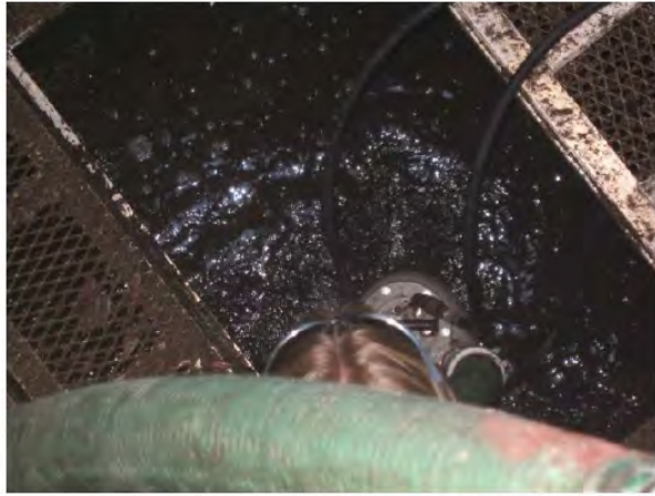
b. Water pumped from sump area
