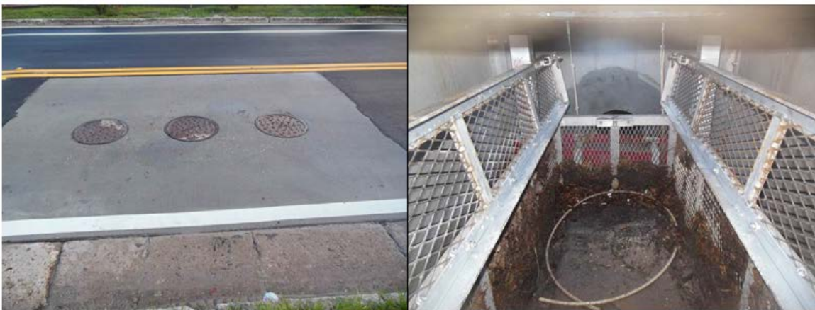
FIGURE 6: CITY OF SANFORD'S NEW BAFFLE BOX INSTALLED ON SANFORD AVENUE
