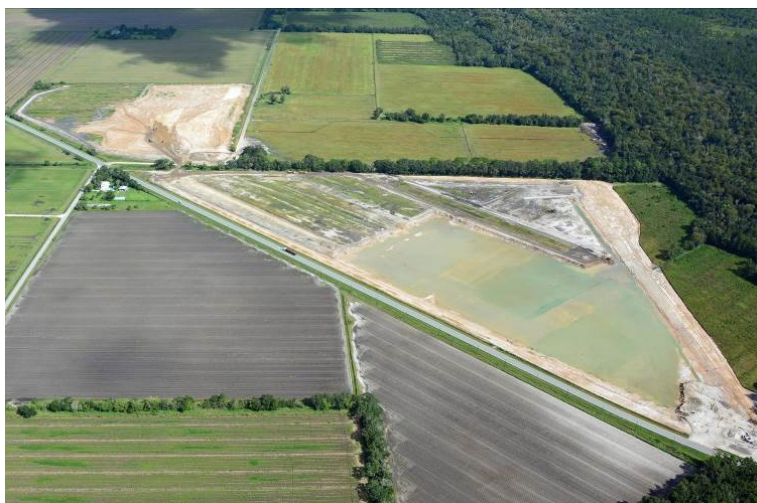
FIGURE 15: ST. JOHNS COUNTY MASTERS TRACT RST FACILITY CONSTRUCTION IN SEPTEMBER 2013
