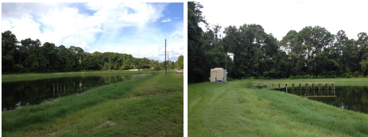
FIGURE 9: NAS JACKSONVILLE REUSE HOLDING POND AND IRRIGATION PUMP STATION
