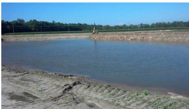
FIGURE 16: ST. JOHNS COUNTY MASTER TRACT RST FACILITY WET DETENTION POND CONSTRUCTION
