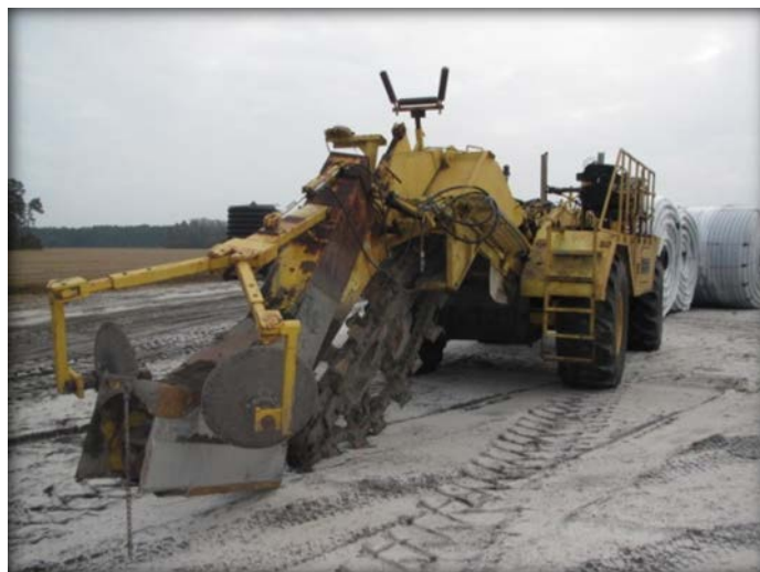
FIGURE 24: INSTALLATION OF IRRIDRAIN SYSTEM
