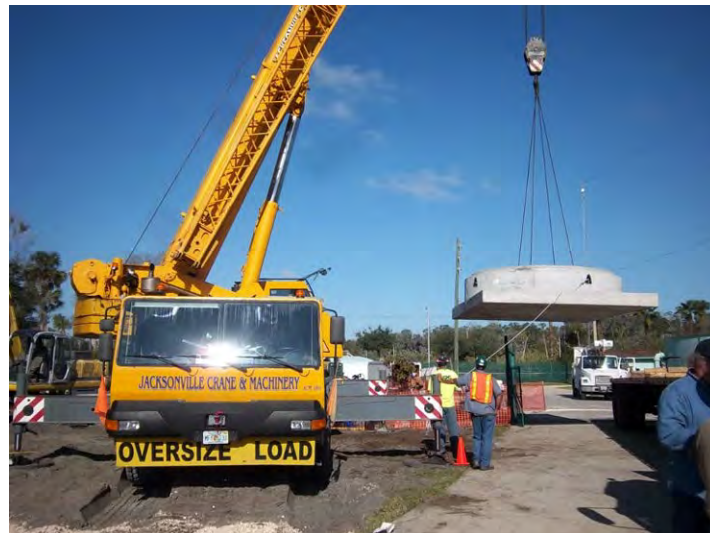
FIGURE 10: LIFT STATION CONSTRUCTION TO TRANSFER FLOWS FROM ATLANTIC BEACH WWTP #2 TO WWTP #1
