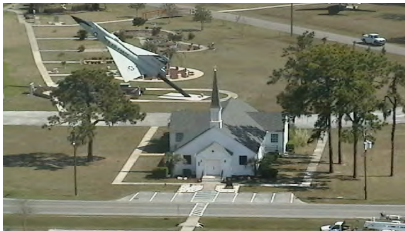
CAMP BLANDING CANTONMENT AVENUE B
