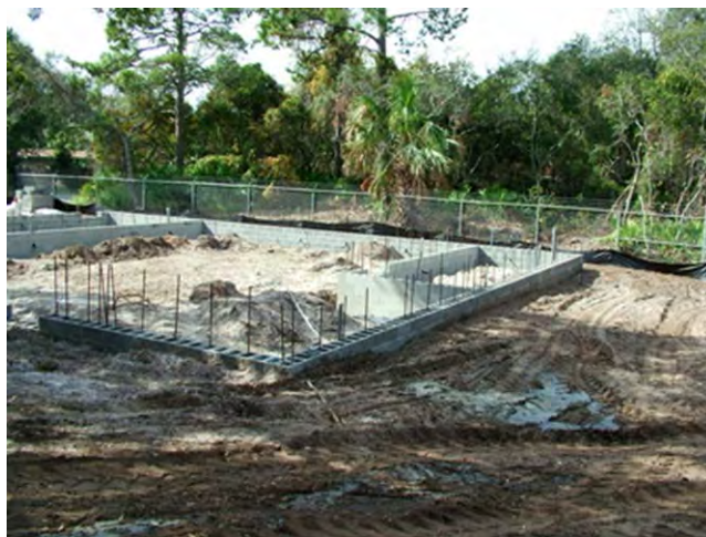
CONSTRUCTING NEW SLUDGE TREATMENT BUILDING WITH CENTRIFUGE
