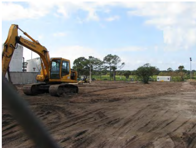
FIGURE 13: BACKFILL OF JACKSONVILLE BEACH OLD WWTP AREA
