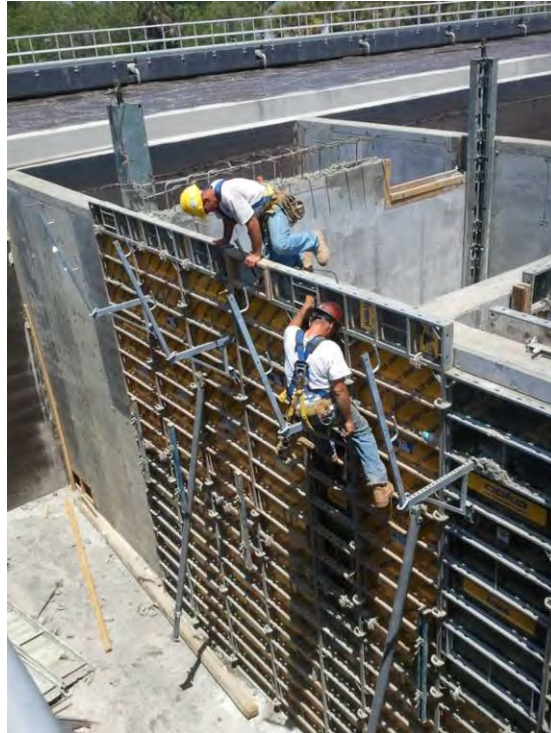
BAFFLE WALLS CONSTRUCTED IN EXISTING AERATION TANKS AT WWTP #1
