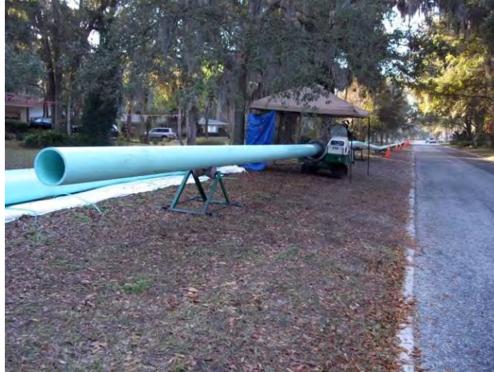
FIGURE 9: DIRECTIONAL DRILLING OF FORCE MAIN FOR ATLANTIC BEACH MAIN WWTP UPGRADE
