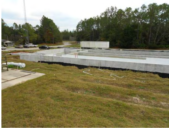
FIGURE 5: PALATKA WWTF UPGRADES
