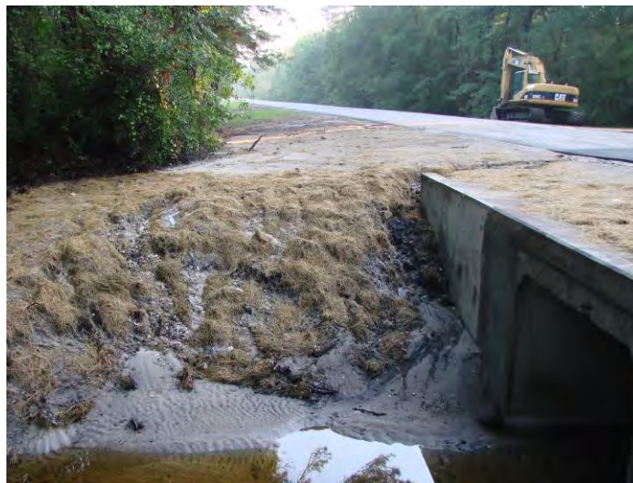
NORTH FORK BLACK CREEK DURING CULVERT REPLACEMENT
