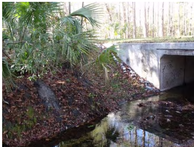
FIGURE 39: CAMP BLANDING NORTH FORK BLACK CREEK AFTER INSTALLATION
