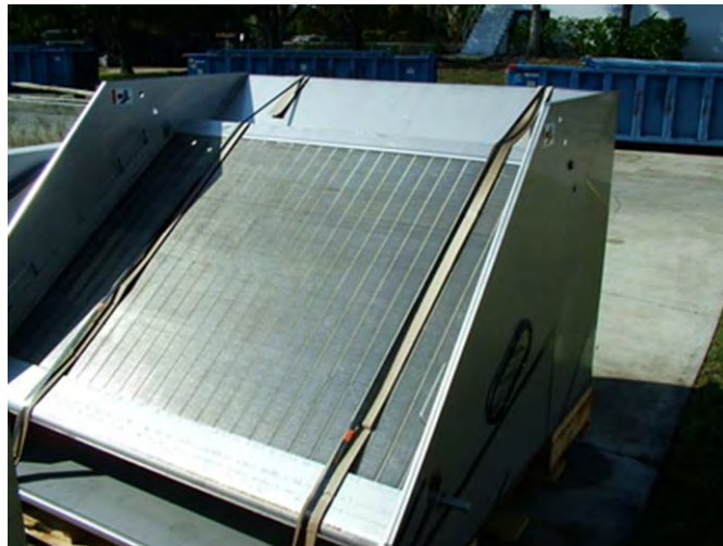
ADDITIONAL STATIC SCREENS INSTALLED AT HEADWORKS
