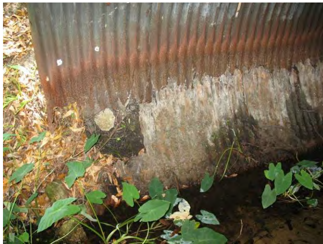
FIGURE 38: CAMP BLANDING NORTH FORK BLACK CREEK CULVERT BEFORE REPLACEMENT
