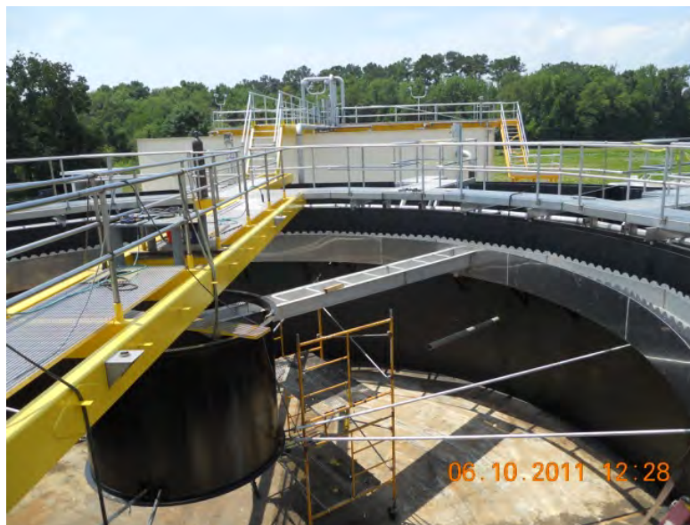
ASH STREET WWTF CLARIFIER #2 UNDER CONSTRUCTION
