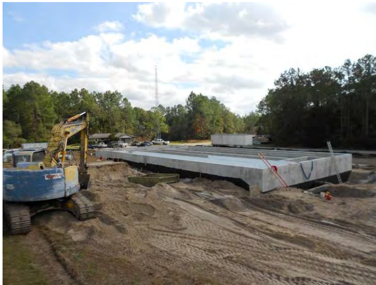
FIGURE 6: PALATKA WWTF UPGRADES
