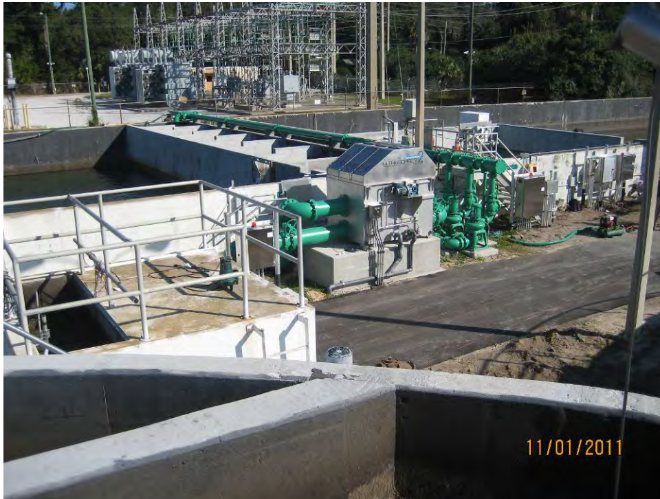
NEPTUNE BEACH UPGRADED WWTf
