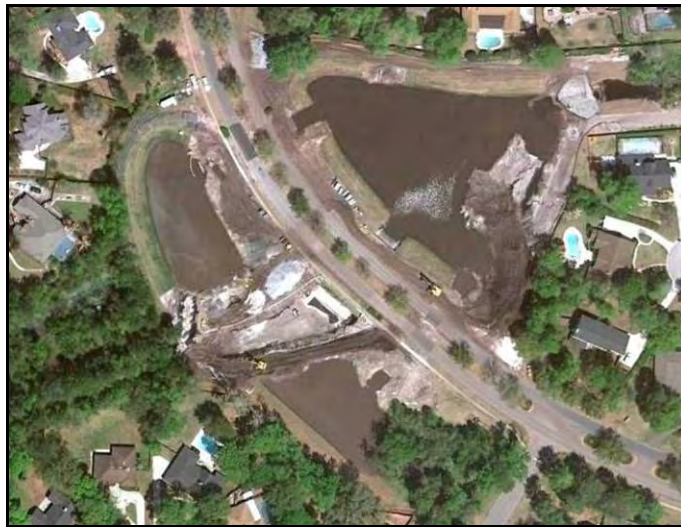
FIGURE 30: CLAY COUNTY LOCH RANE STORMWATER IMPROVEMENTS NEAR COMPLETION IN SPRING 2010
