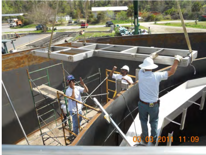
ASH STREET WWTF STAINLESS STEEL BRIDGEWORK FOR INVENT MIXER-AERATORS DURING PHASE 2 CONVERSION
