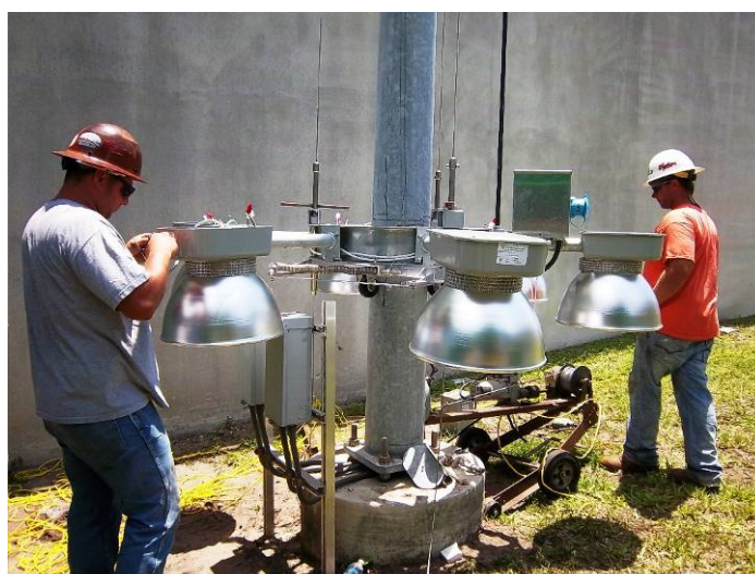
YARD LIGHTING REPLACED WITH ENERGY EFFICIENT LIGHTING
