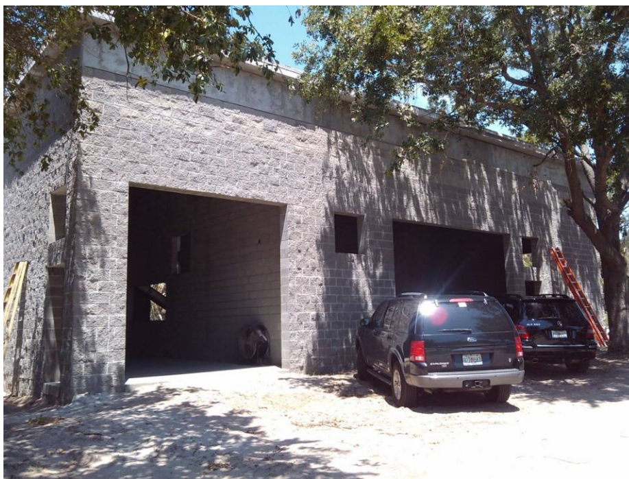
NEW SLUDGE TREATMENT BUILDING CONSTRUCTED
