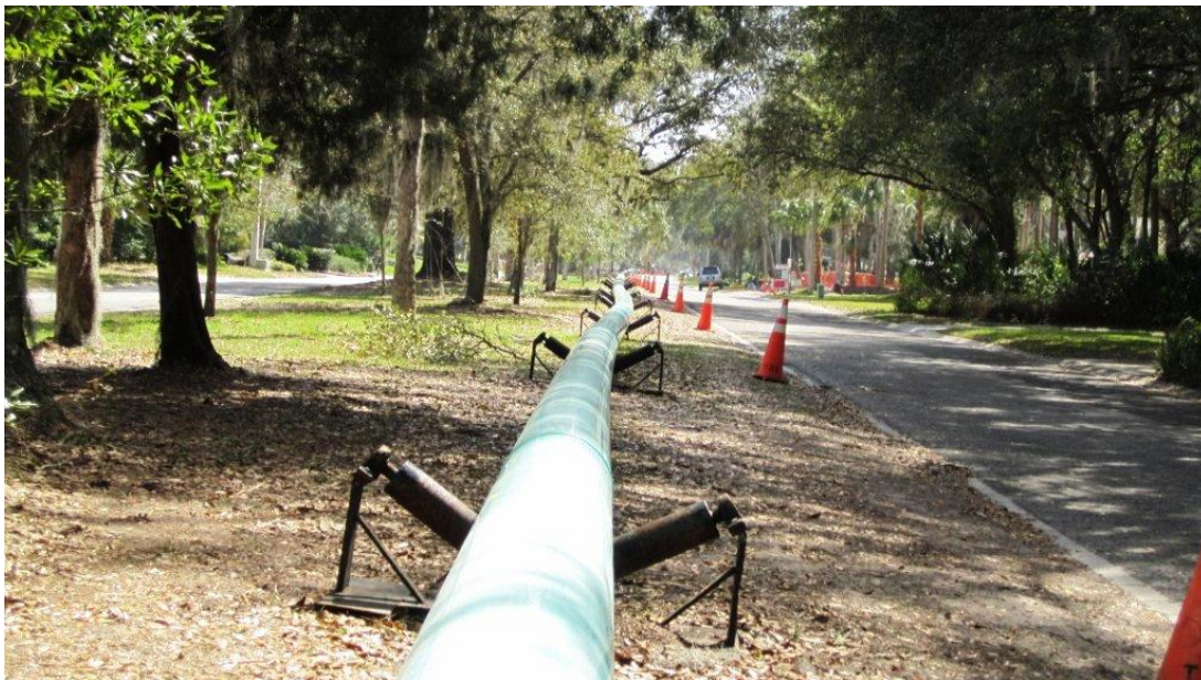
DIRECTIONAL DRILLING USED TO INSTALL MUCH OF THE FORCE MAIN FROM NEW MASTER LIFT STATION TO WWTP #1
