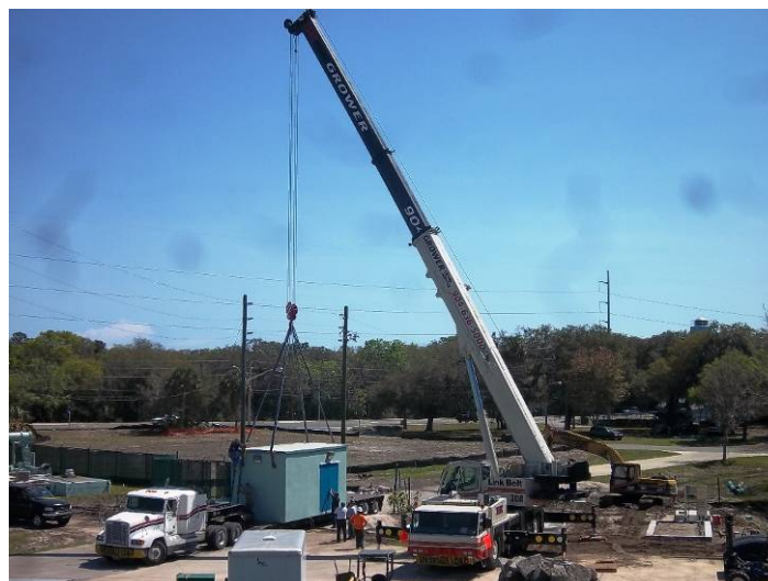
SETTING ELECTRICAL BUILDING FOR NEW MASTER LIFT STATION AT WWTP #2
