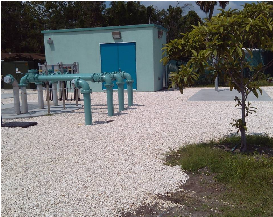
NEW MASTER LIFT STATION LOCATED AT FORMER WWTP #2 SITE
