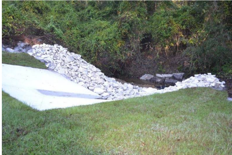
FIGURE 25: CAMP BLANDING WWTP NEW EROSION CONTROL STRUCTURE
